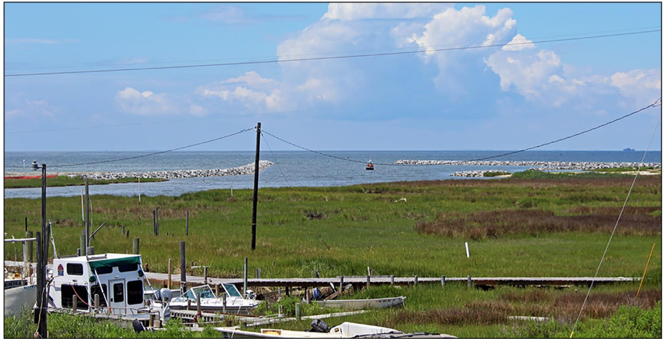
Figure 4: Completed Rhodes Point Jetty, Smith Island
