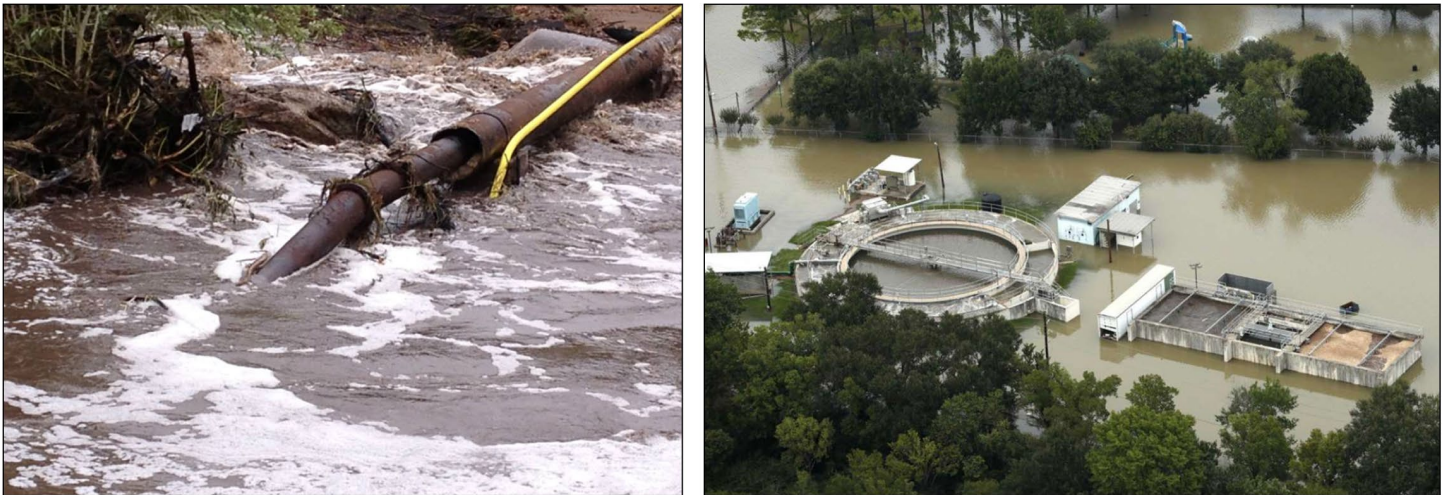
Figure 3: Upper Thompson Sanitation District's 8-Inch Main Collapse during 2013 Flood and Houston Water's Flooded Wastewater Treatment Plant during Hurricane Harvey, 2017
