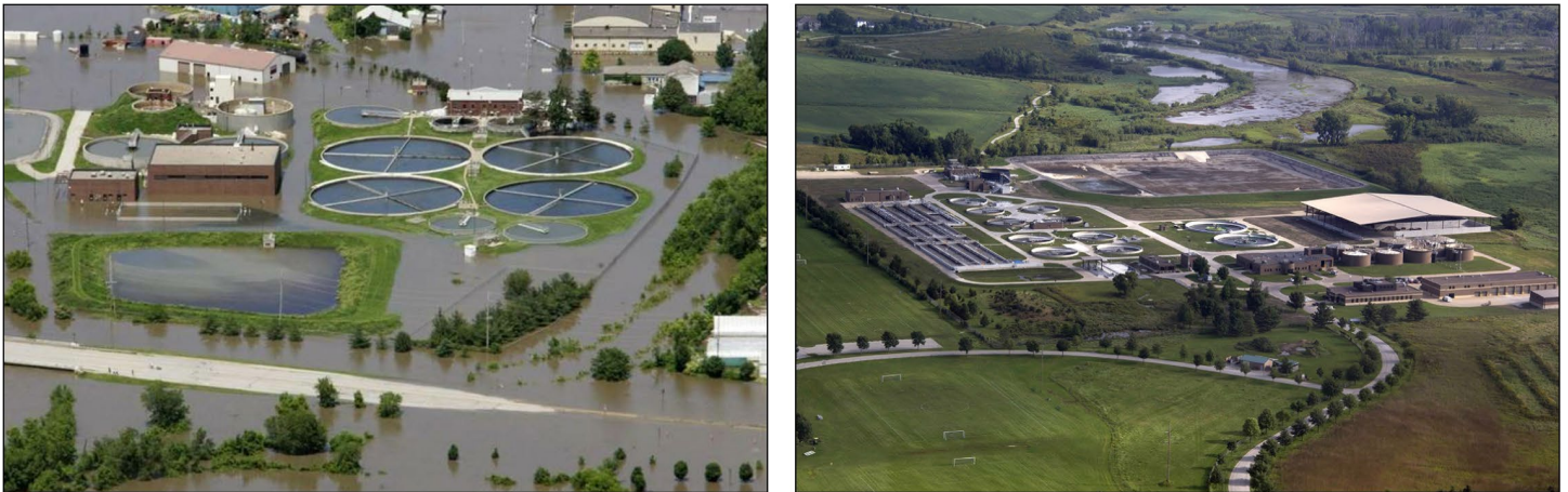
Figure 5: Relocation of Iowa City's North Wastewater Treatment Facility Because of 2008 Flooding
