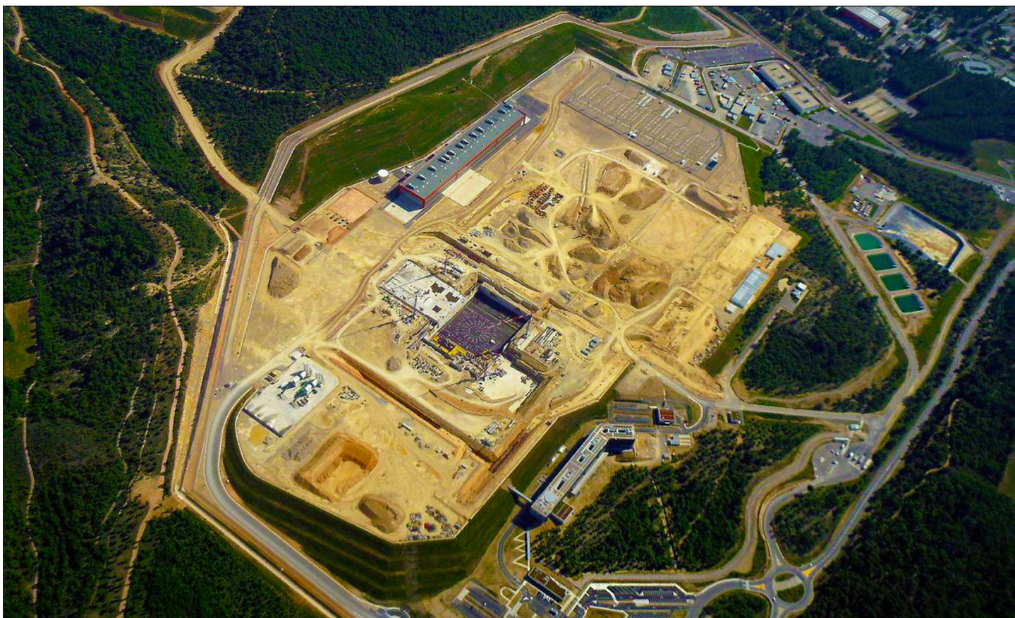
Figure 2: Aerial View of Construction Progress at the ITER Site as of June 2013
