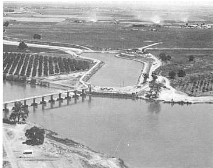
Red Bluff Diversion Dam, a feature of the Central Valley Project in California. This structure illustrates the complicated operations often encountered at irrigation headworks. The facility includes fish diverters and ladders, a sedimentation basin and spawning bed, and the diversion works for the Tehama-Colusa Canal, all of which require well coordinated operation. Photo P-602-200-5667 NA
