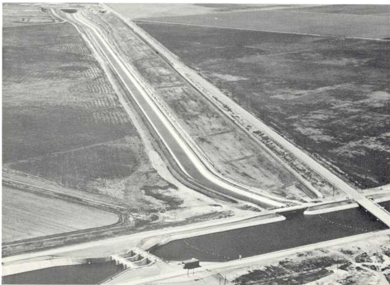
Aerial view of the intake channel to the Pleasant Valley Pumping Plant, a major turnout on the San Luis Canal a few miles from Coalinga, California. Photo P805-200-587 NA
