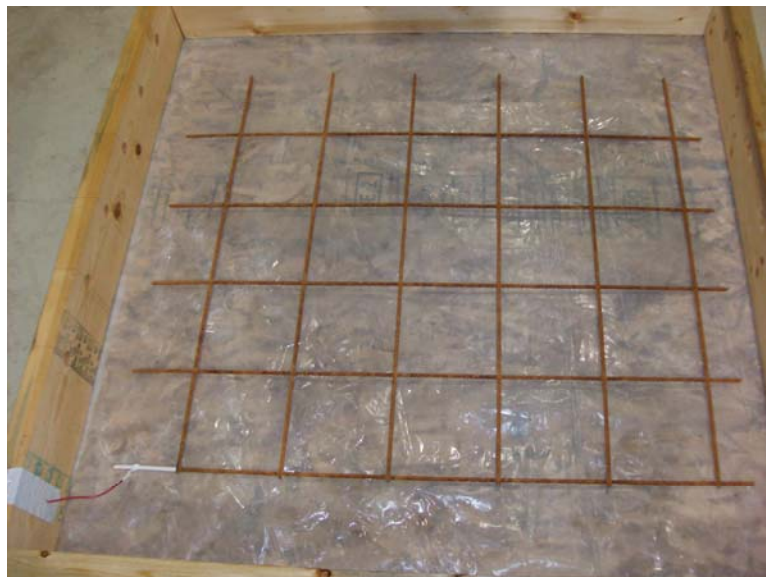
Figure 69 - Weld Wire Fabric Located in Bottom of Form
