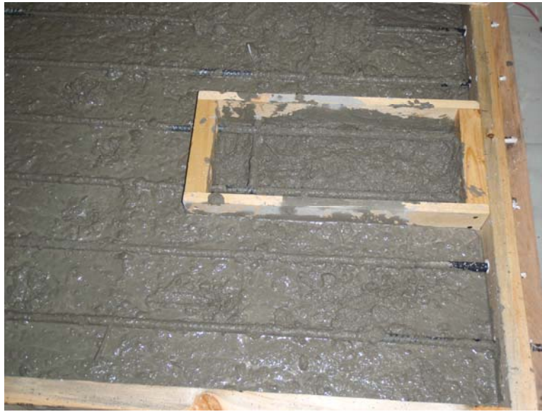
Figure 79 – Construction with block out for modified concrete hotspot
