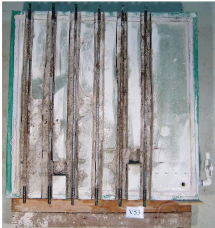
Figure 134 – Bird's eye view of exposed rebar positioned in slab
