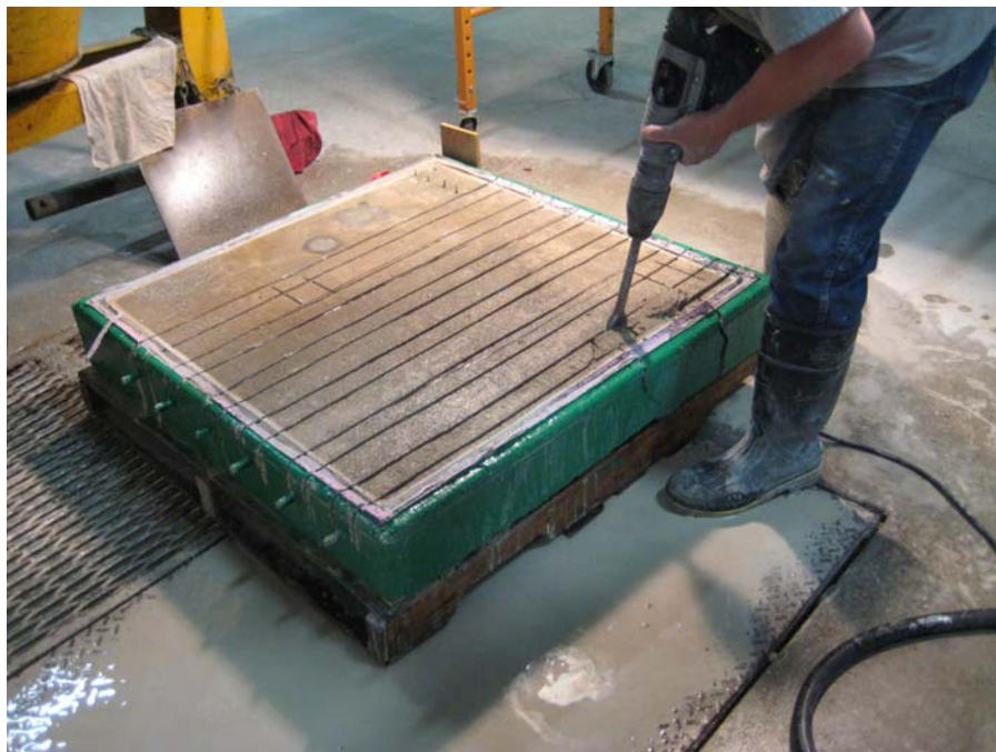
Figure 131 – Chip away and remove concrete adjacent to rebar
