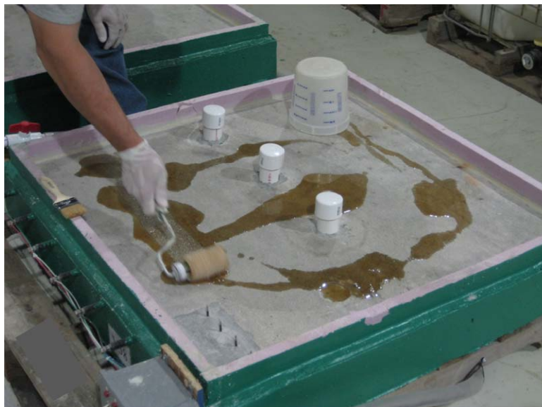
Figure 110 – Application of primer
