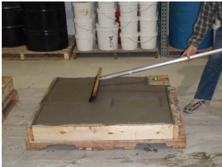
Figure 76 - Broom Finish Application
