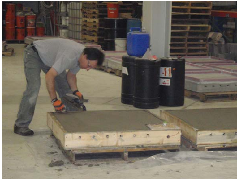
Figure 75 - Installing Tooled Edge
