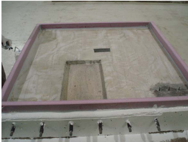
Figure 87 – Installation of Closed Cell Insulation to Form Ponding Dam
