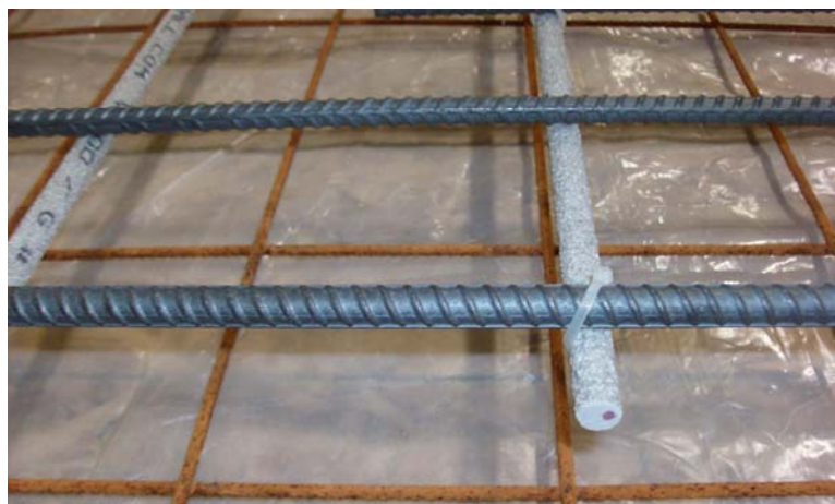
Figure 67 - GFRP Reinforcement Bar
