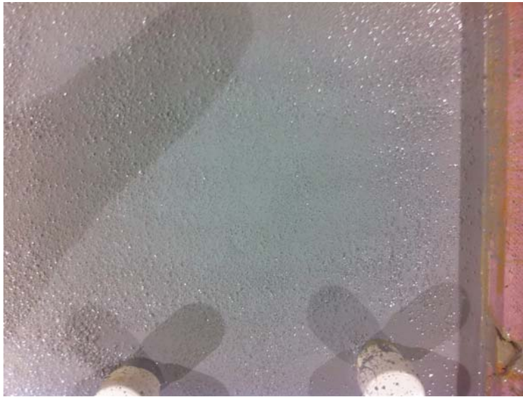
Figure 117 – Completed epoxy coating surface
