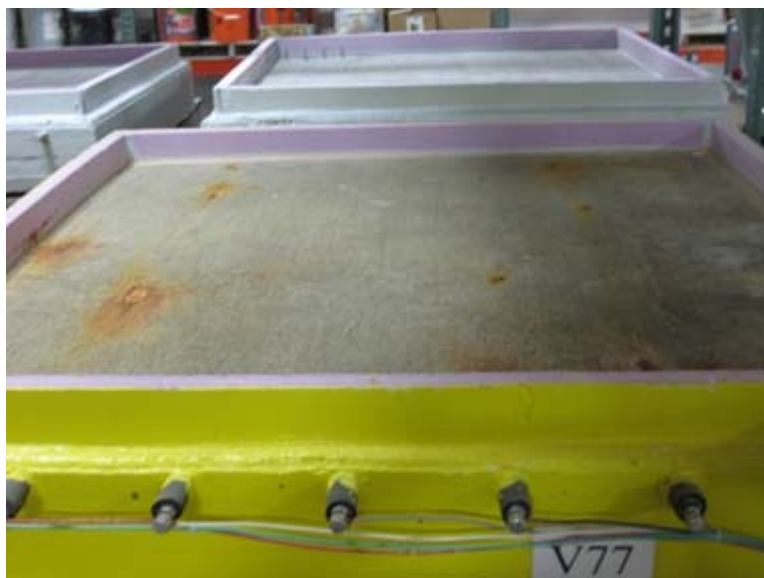
Figure 52 – Slab with visual corrosion damage on surface (0.75-inch cover, Batch #4, Slab 77)
