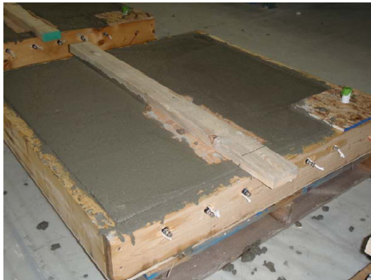
Figure 78 – Construction of depressed cover hotspot
