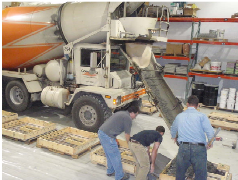
Figure 72 – Concrete placement in forms
