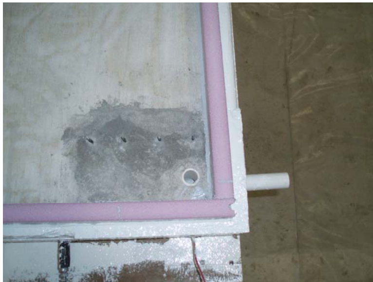
Figure 94 - PVC Piping Installed to Provide Drainage for Ponding Solution
