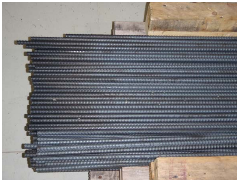
Figure 61 – Wire brushed reinforcing bars
