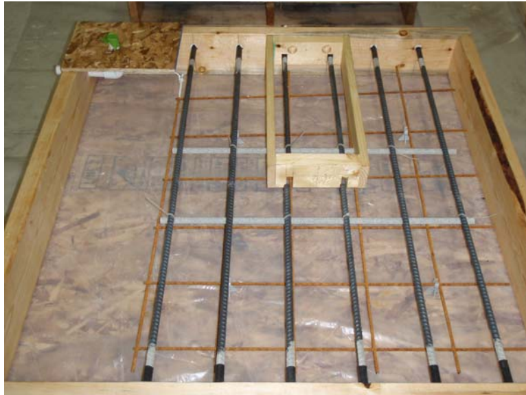
Figure 70 – Hotspot Repair Form and Reinforcement Configuration
