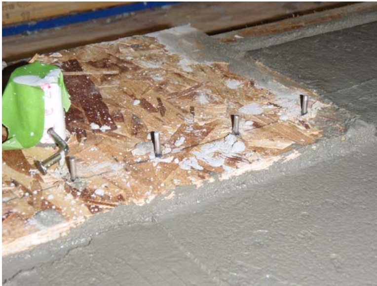
Figure 83 – Resistivity measurement pins inserted during concrete finishing
