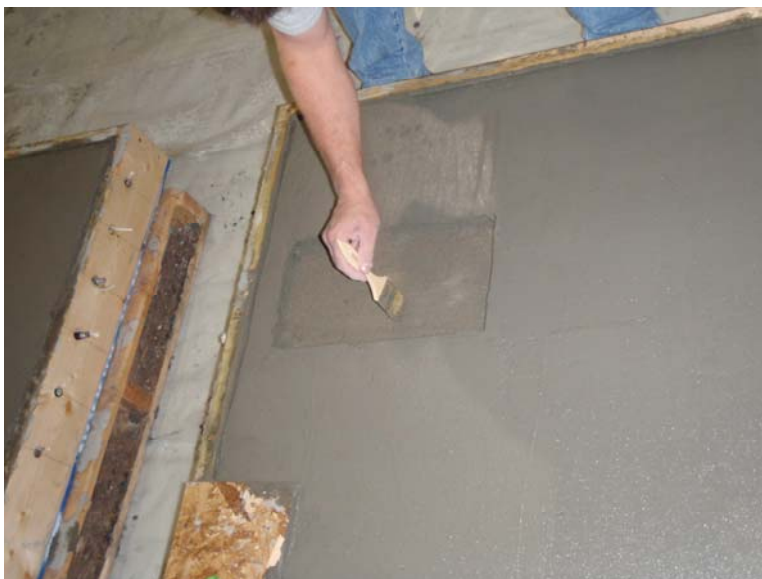
Figure 77 - Broom Finish Application to Hotspot
