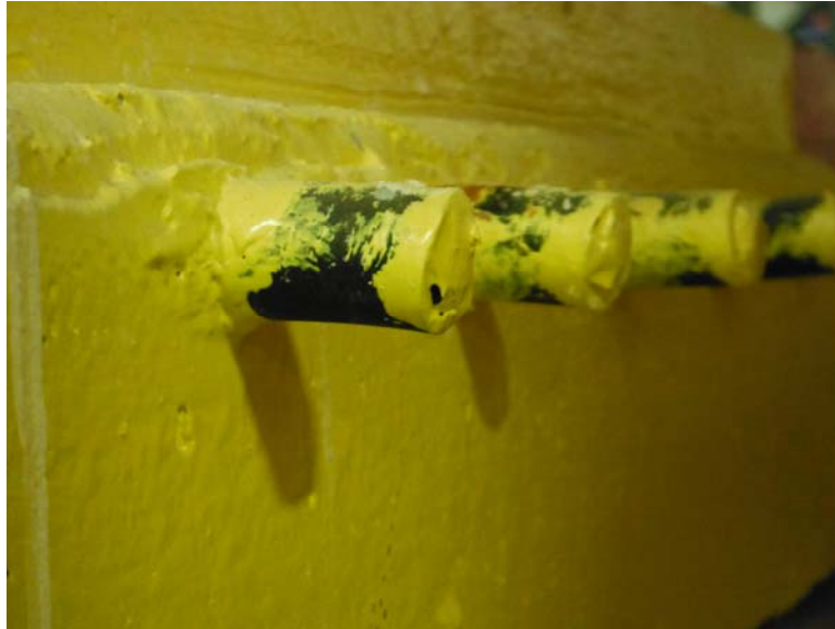
Figure 65 – Photograph of batch #4 reinforcing bar end treatment
