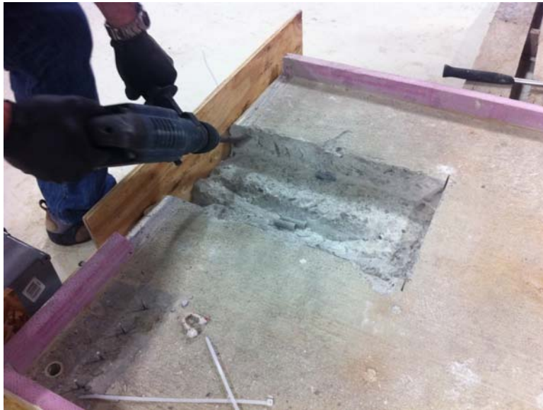
Figure 120 – Roughen saw cut edges
