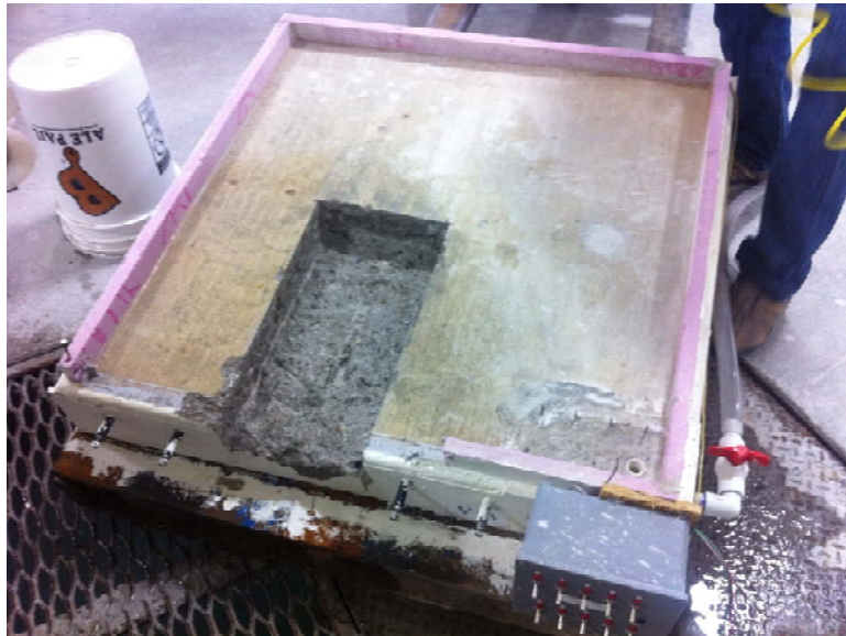
Figure 122 – Cleaned repair area
