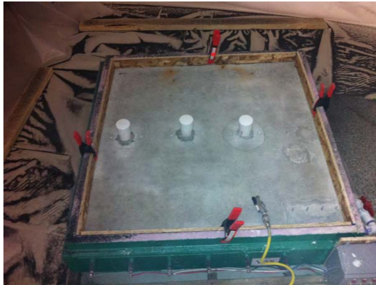
Figure 109 – Shot blasting slab surface
