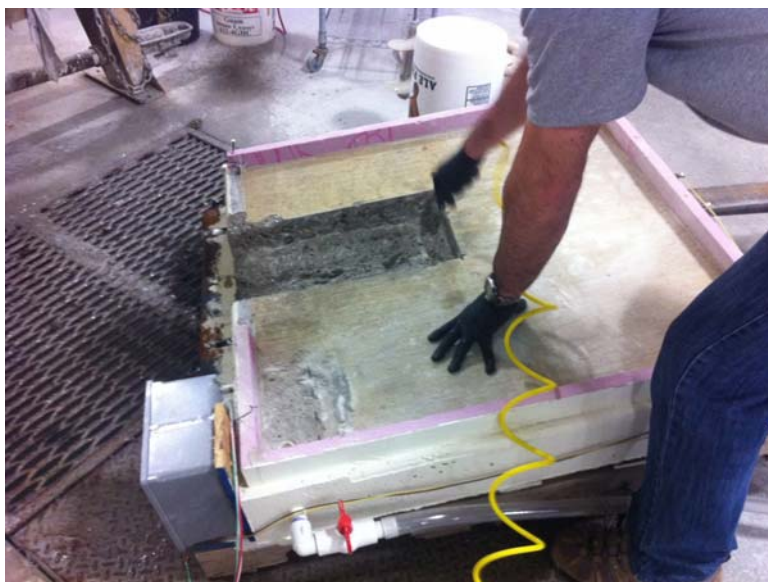
Figure 121 – Clean and blow out repair area
