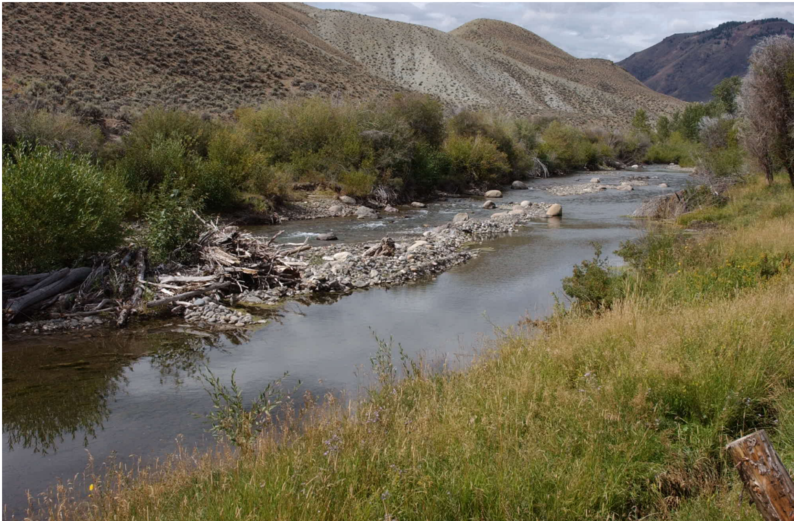
Figure 4.1 – Looking upstream at the berm that was pushed up on a regular basis to guide flow to the irrigation diversion prior to installation of the A-weir.
