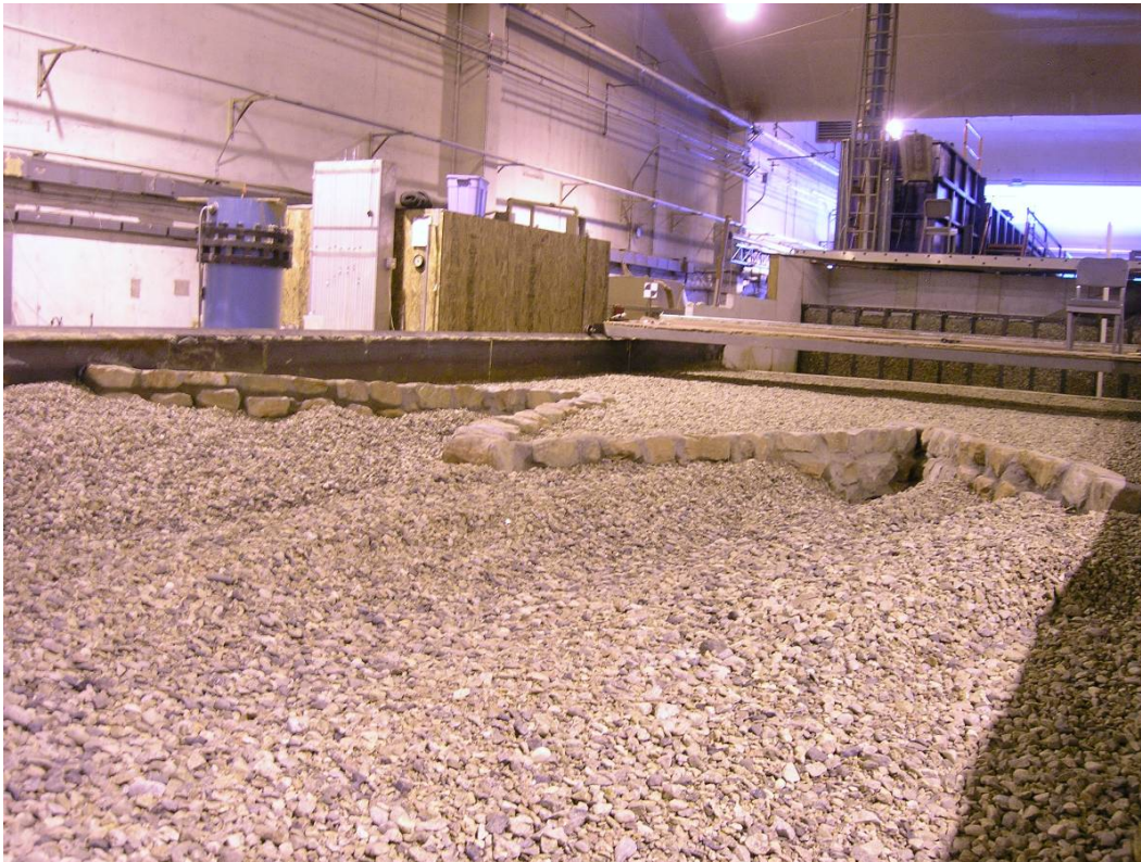
Figure 5.1. Example of a W-weir constructed at the CSU Hydraulics Laboratory, showing Test 50.
