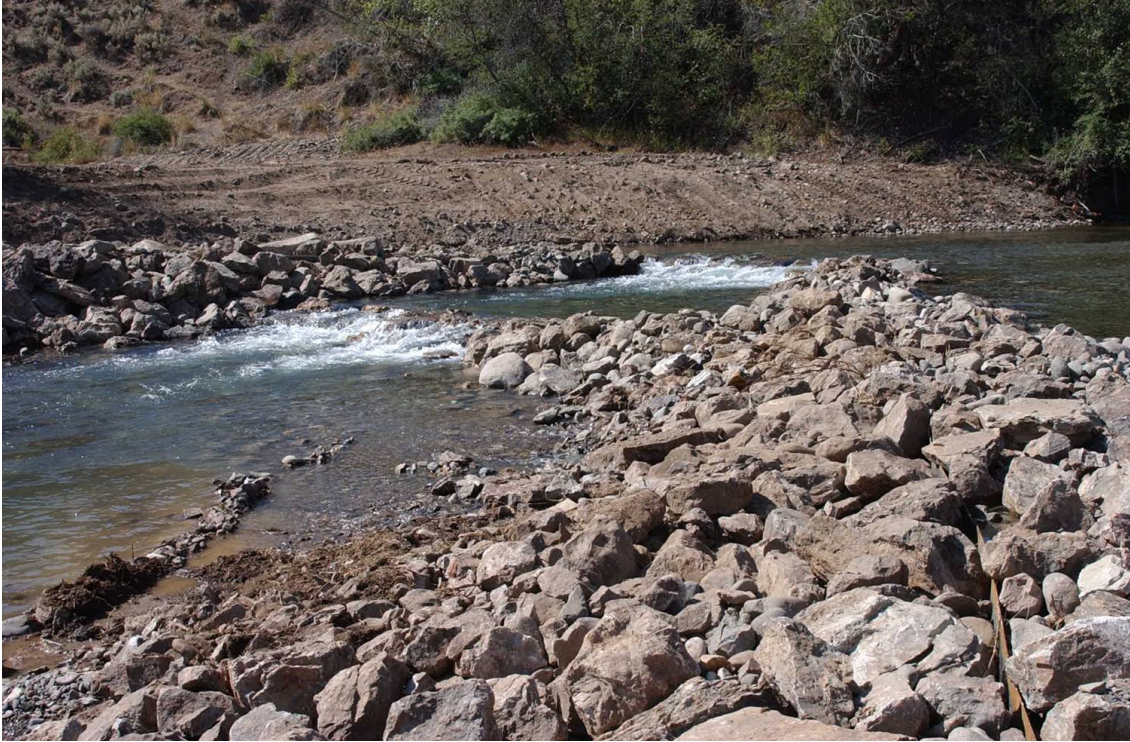
Figure 4.2 – Site post construction in August 2003, looking upstream.
