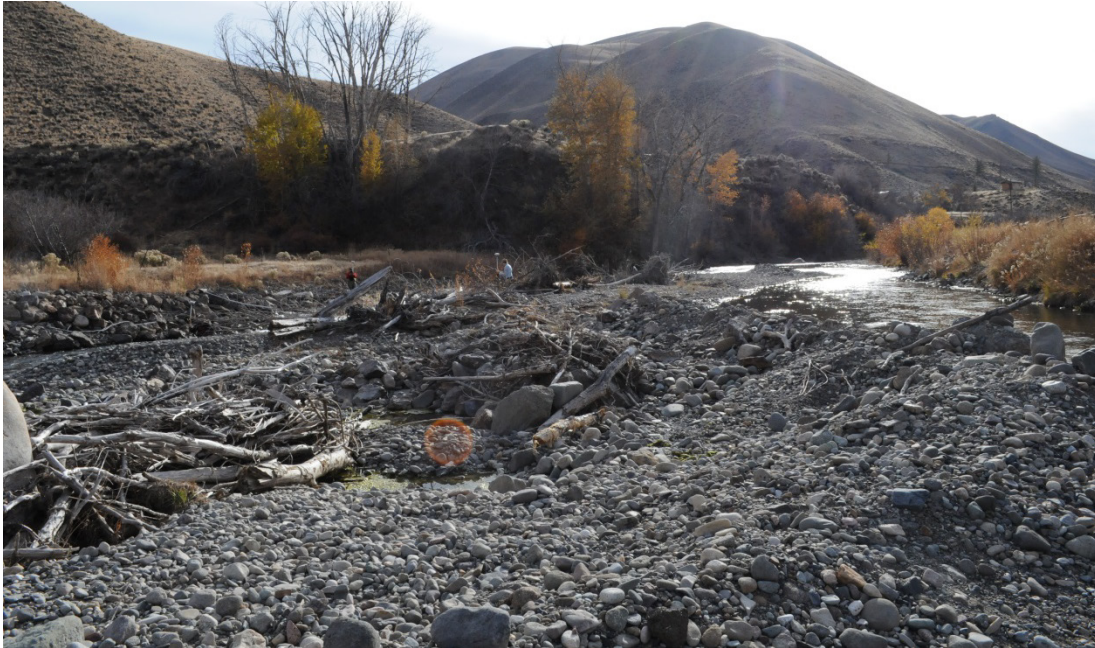
Figure 4.6 – Looking upstream from where the left arm of the structure lies buried under large gravel bar and large woody material (October 2008).
