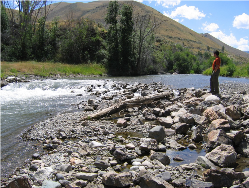
Figure 4.3 – July 2005. Note depositional zone upstream from structure on right side of the photo (left bank).
