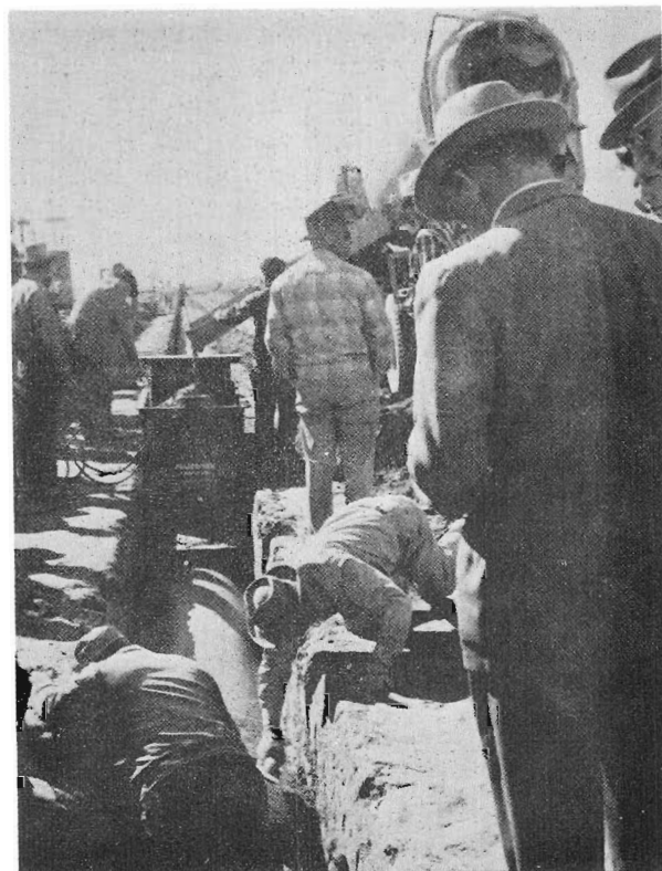
Figure 65.—A monolithic unreinforced concrete pipe machine in operation in an excavated trench. CH-357-62.
