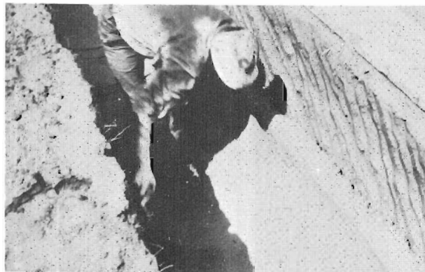
Figure 62.—Placing lower portion of unreinforced cast-in-place concrete pipe. P214-D-33702, 33705, 33706.
