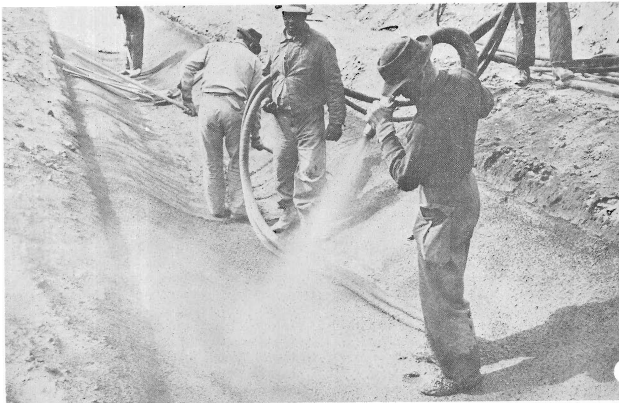
Figure 28.—Placing shotcrete lining in a small canal. C-7330-3.
