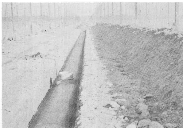
Figure 66.—A completed section of monolithic unreinforced concrete pipe. CH-357-17.
