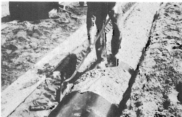
Figure 63.—Placing upper portion of unreinforced cast-in-place concrete pipe. P214-D-33704, 33703.
