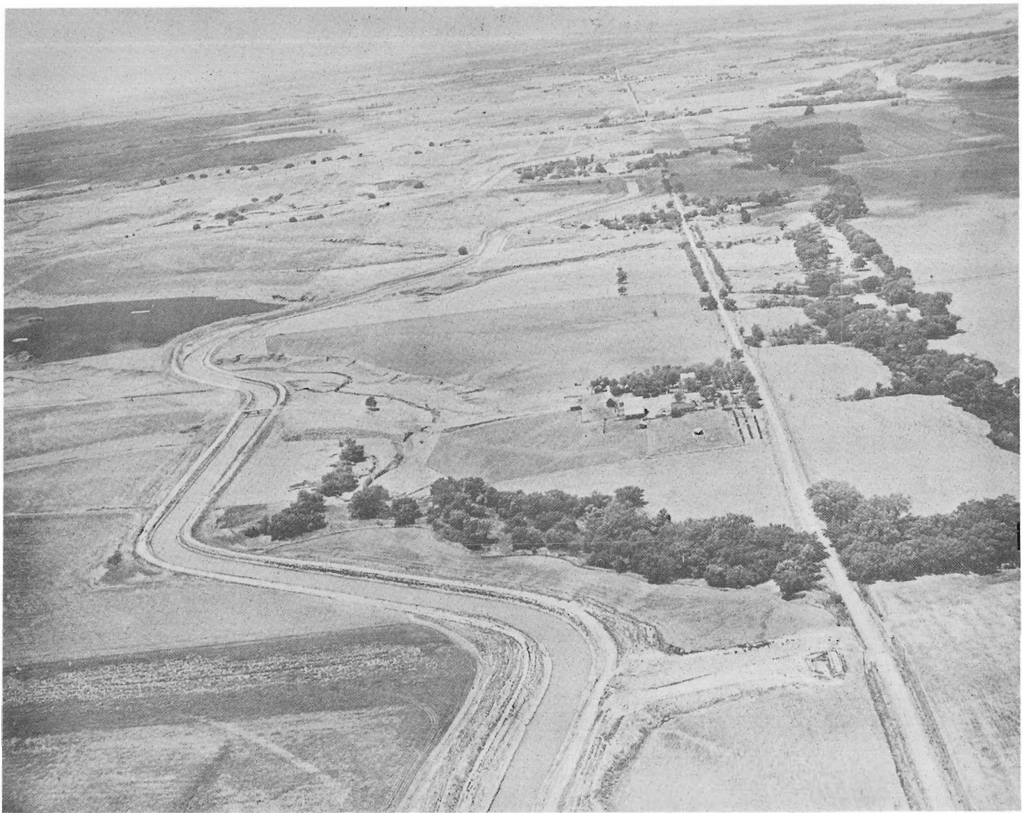
Frontispiece. —View of Courtland Canal, Bostwick division, Missouri River Basin project, showing compacted-earth lining in the foreground. 271-701-2200.
