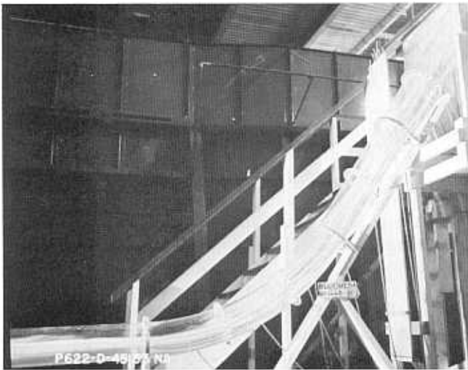
B. Inclined tunnel. P622-D-45163NA
