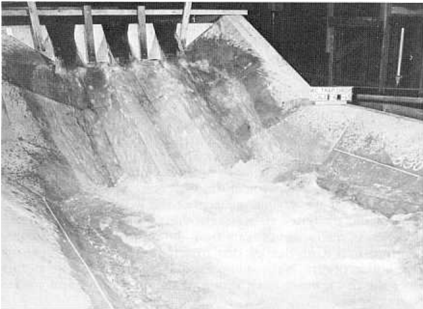
Figure 6-2.—Check and chute for trapezoidal canal. P801-D-79220
