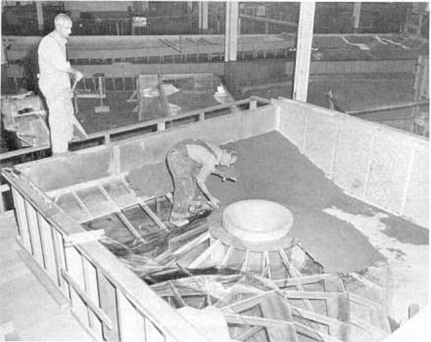
Figure 4-1.—Model of morning glory spillway under construction P801-D-79229
