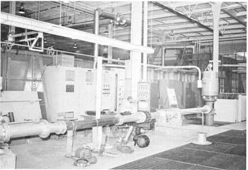
Figure 9-12.—Investigation of butterfly valve opening and closing characteristics. P801-D-79245
