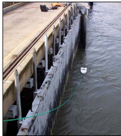
Figure 34. Positioning the ADP in front of the bypass intake.
