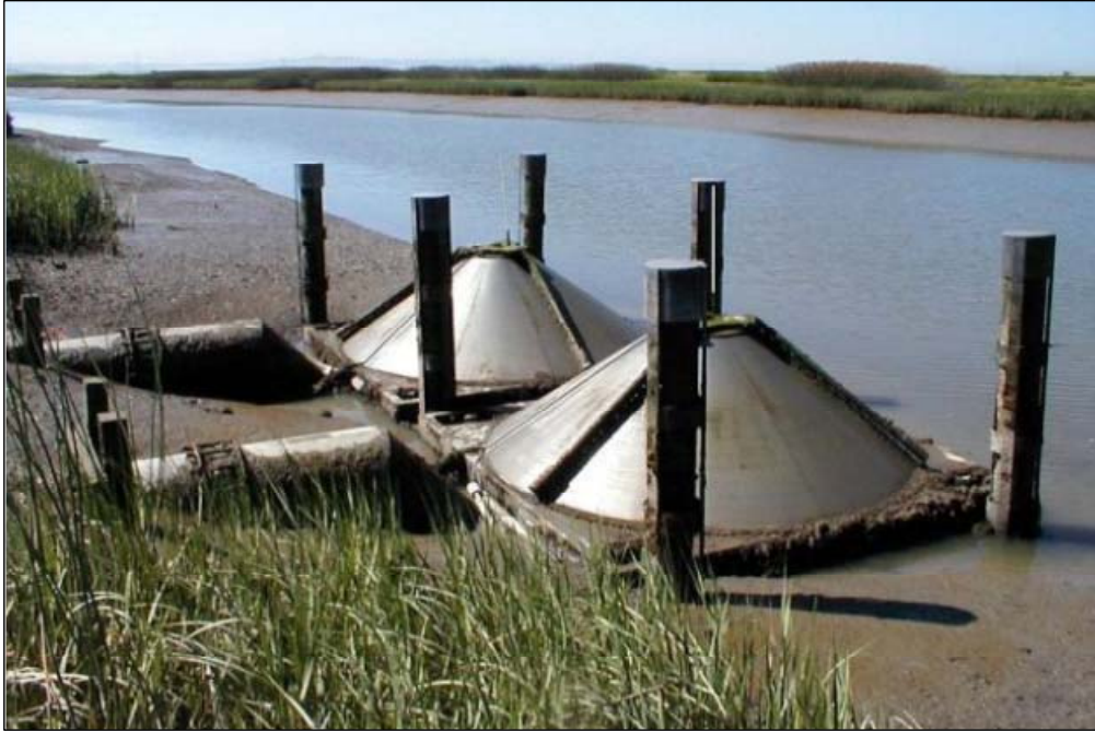
Figure 8. Cone screen installed by Intake Screens, Inc. Cone screens are typically used in shallow estuaries or tidally influenced areas (photo courtesy of Intake Screens, Inc.)
