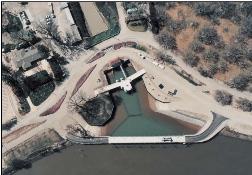
Figure 2. Flat plate screens installed at Wilkins Slough Pumping Plant on the Sacramento River (Reclamation District No. 108). On-river fish screens are common for large diversions.
