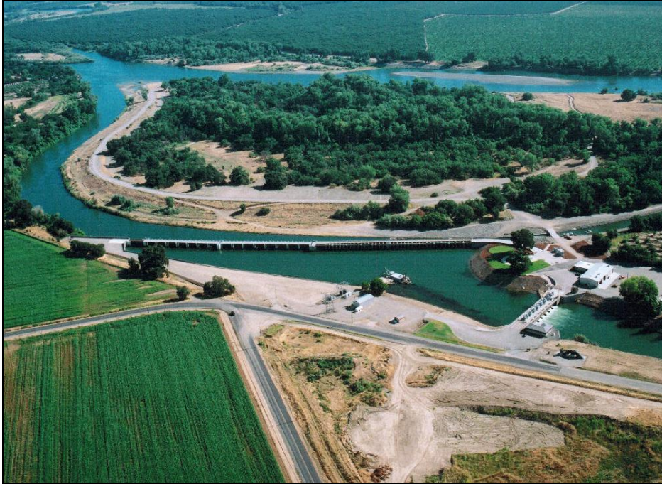
Figure 23. GCID's Hamilton City diversion facilities located in an oxbow along the Sacramento River.
