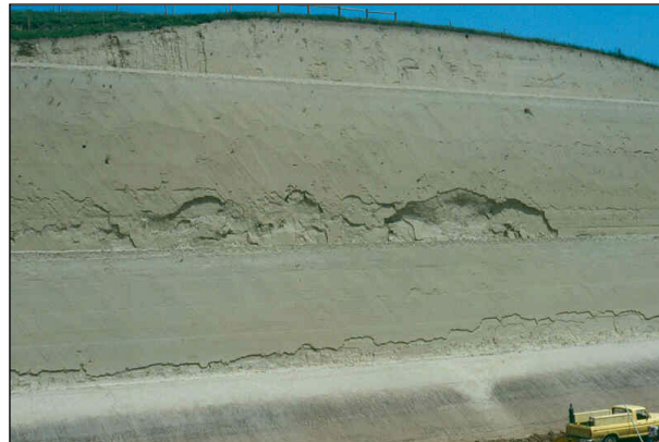
Figure 62. —Popouts in a \frac{3}{4} :1 cut in Loess, caused by weak material.
