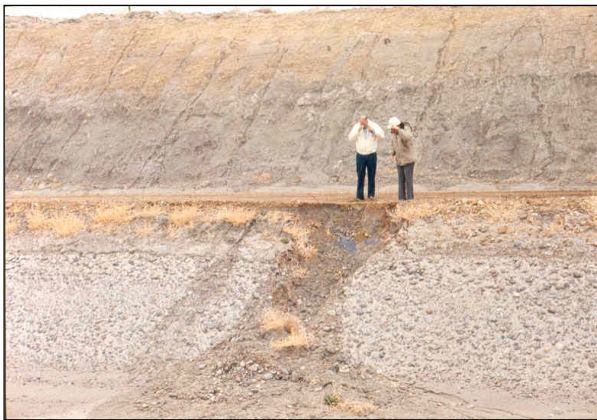
Figure 56. —Gravel-lined canal—water drained down an open slope, across a road, and along the lining under the gravel.
