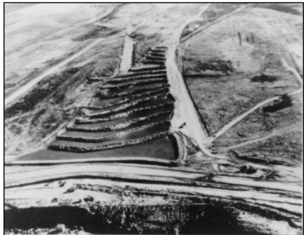
Figure 49. —Ponding dry foundation of Trenton Dam in Nebraska [1].
