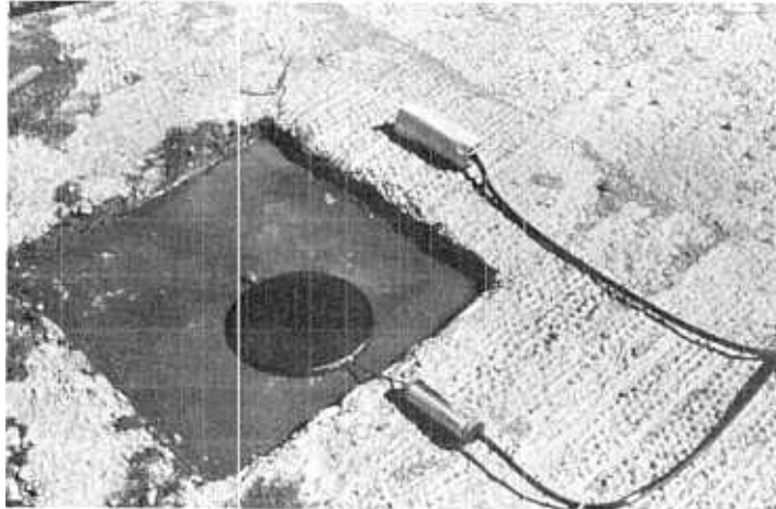
Figure 2-34.—Pneumatic total pressure cell installation. P801-D-81013.
