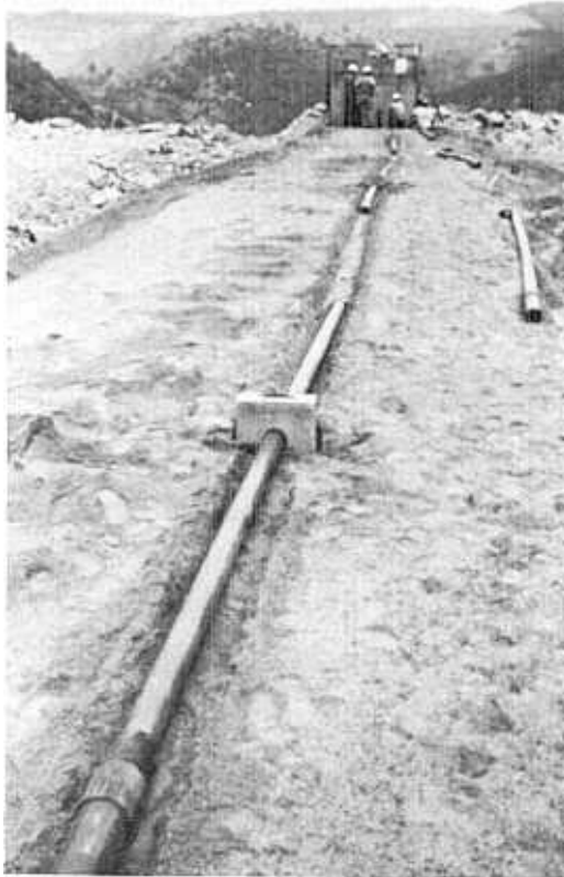
Figure 4-28.—Typical radiosonde installation. P801-D-81023.
