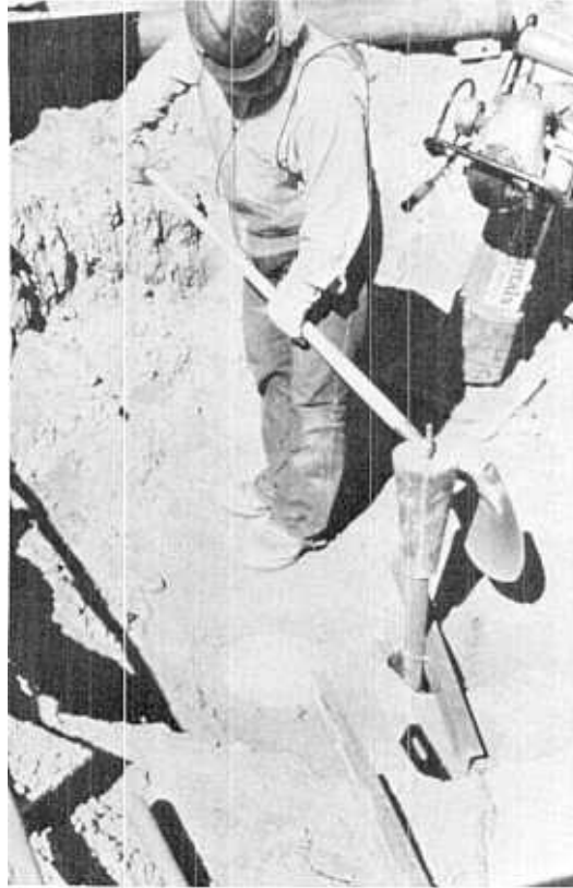
Figure 4-2.—Installation of internal vertical movement device. P801-D-81017.
