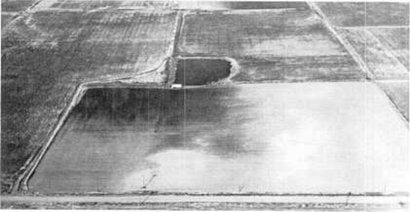
Before drain construction. 10-27-66. P222-D-77008.
