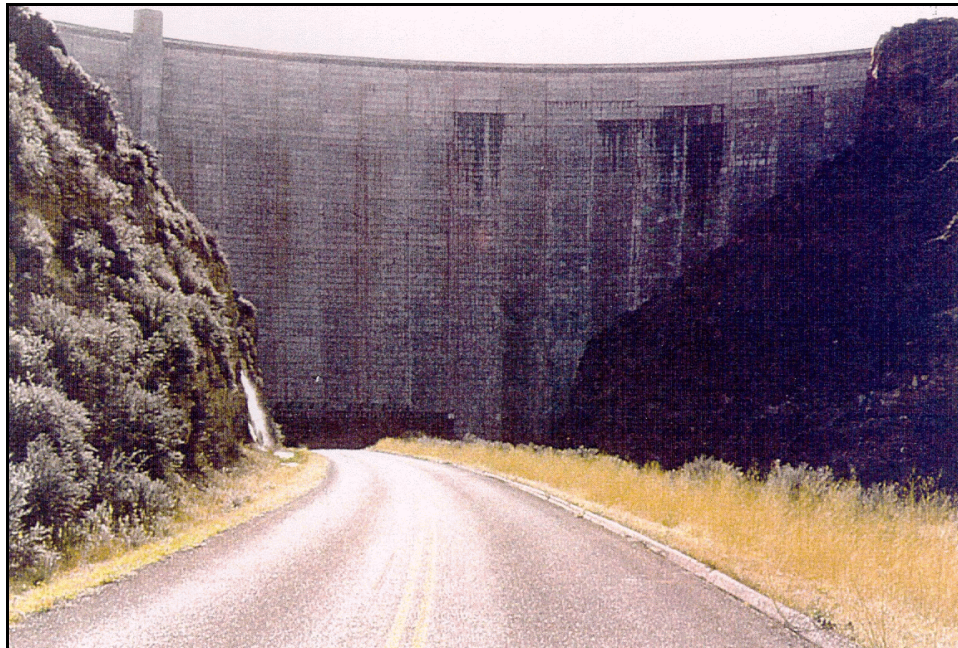
Figure 1. —View of the downstream face of the dam from the access road along the river.
