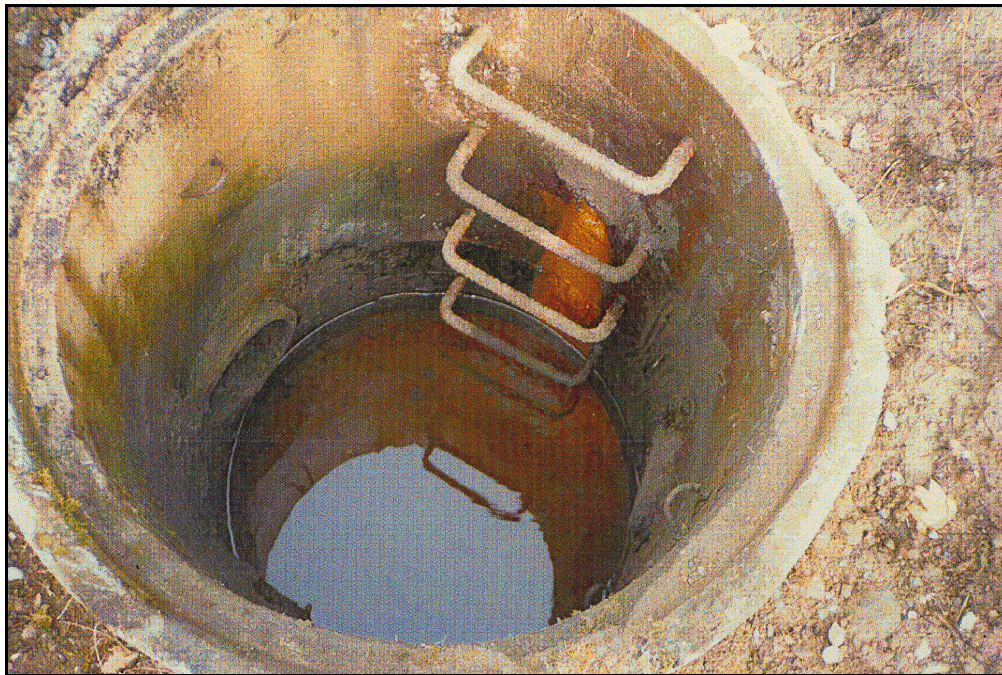
Figure 70.—Typical inspection well used to gain access to outfall pipes.
