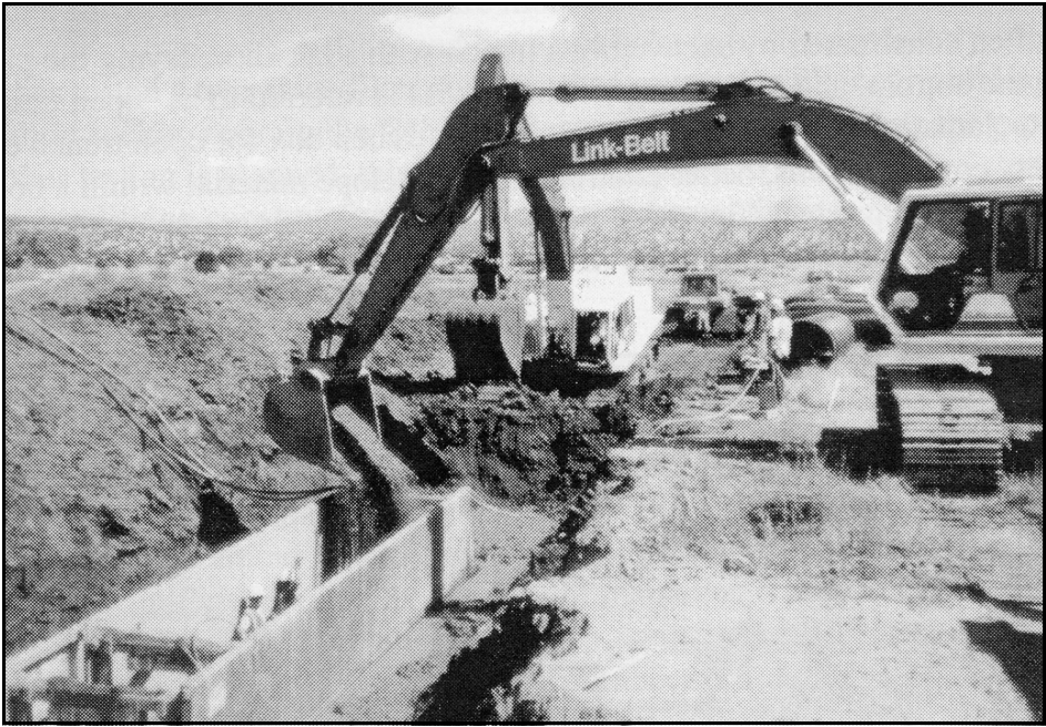
Figure 47.—Open trench excavation with a trench box.
