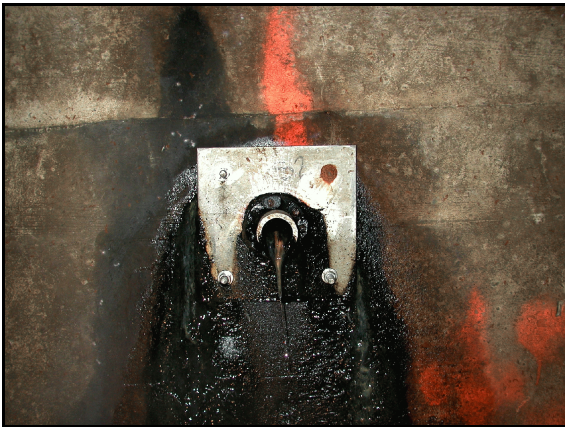
Figure 43. —The weep shows an example of a sulfate (black) related biofilm
