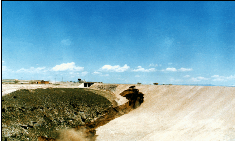
Figure 3.—Piping through the embankment leads to the failure of a dam.
