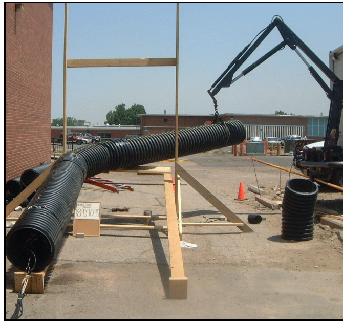
Figure 3. —Apparatus used for performance testing of remotely controlled video inspection equipment within HDPE pipe.
