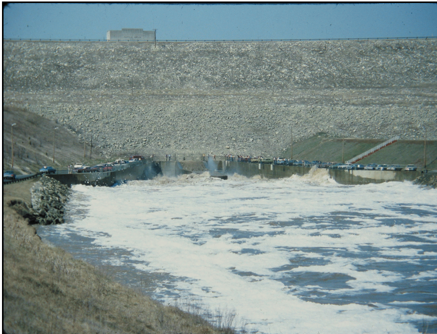
Figure 86.—Tuttle Creek Dam.
