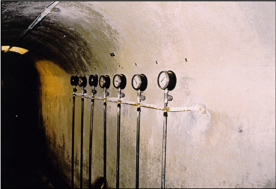
Figure 16.—Uplift pressure gauge readings are recorded before and after cleaning.
