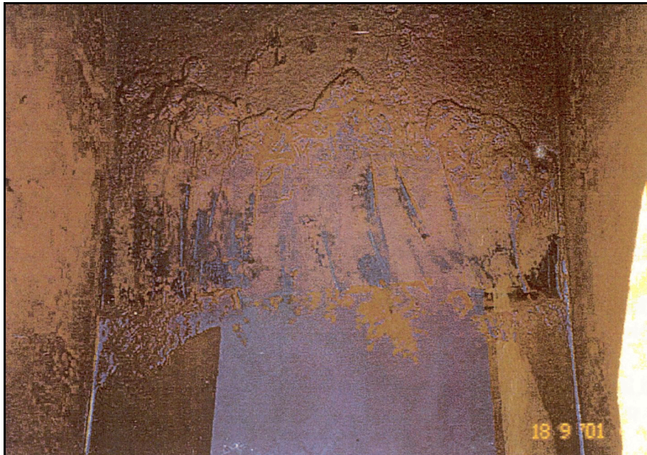
Figure 94. —Sediment sump for SM-D11 and -D12 showing fines that accumulated in one season.
