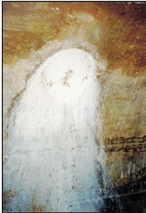
Figure 111. —Calcium carbonate deposit.
