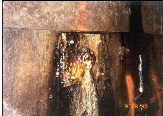
Figure 45. —The weep hole shows an example of sulfur (yellow) and phosphorous (white) related biofilm.
