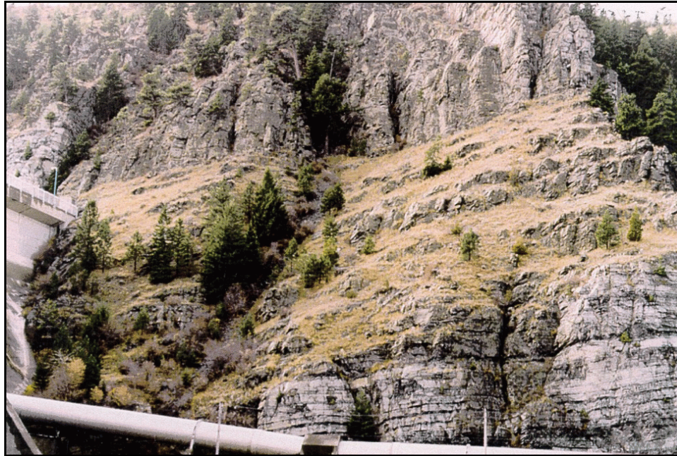
Figure 11. —Empire Shale in the left abutment downstream from the dam.
