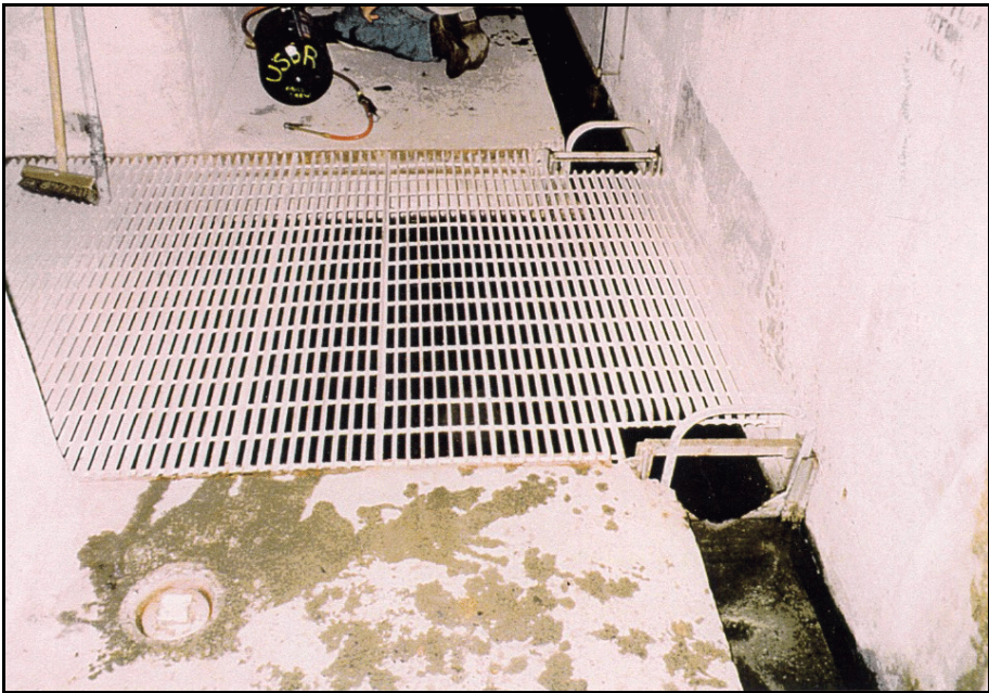
Figure 15.—Weir readings are recorded before and after cleaning.
