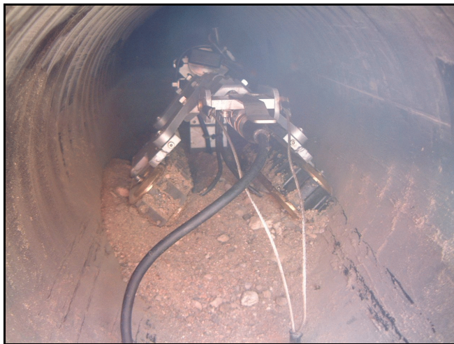
Figure 26. —Example of the gravel invert condition.
