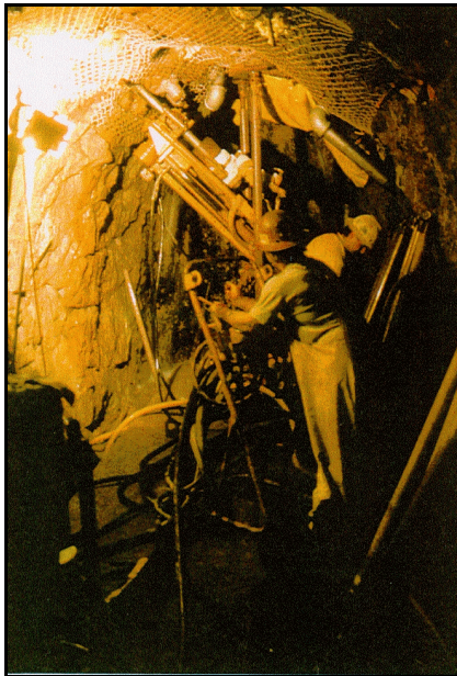
Figure 45. —Views of rotary drilling operations to install high-angle drain holes in bedrock in a drainage adit in the downstream right abutment of Horse Mesa Dam, Arizona. The drill rig is a Craelius Diamec 260. The drill is mounted on a stand when drilling high-angle drain holes.
