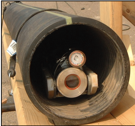
Figure 15. —The MiniTrac system inside an 8-in. diameter pipe.
