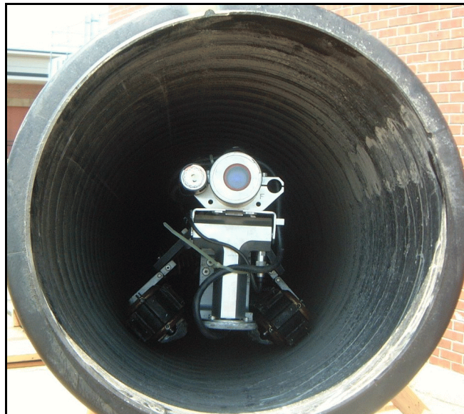
Figure 24. —Example of the dry invert condition.
