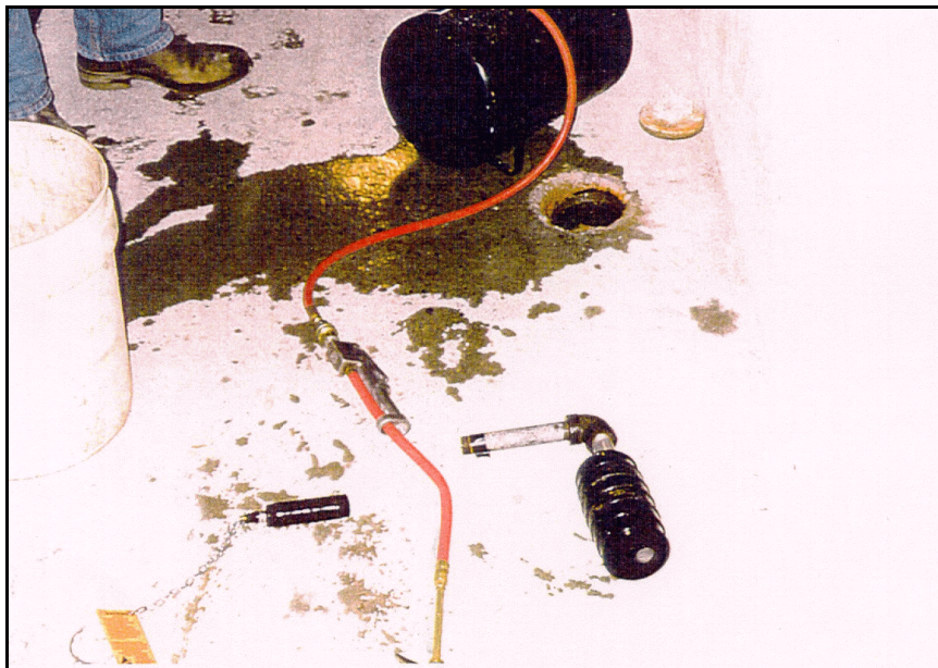
Figure 39. —Portable air tank and pneumatic packers to take before and after cleanout drain flow measurements. The small packer closes the end of the lateral discharge pipe, and the larger packer with the elbow pipe extension goes in at the top of the drain.
