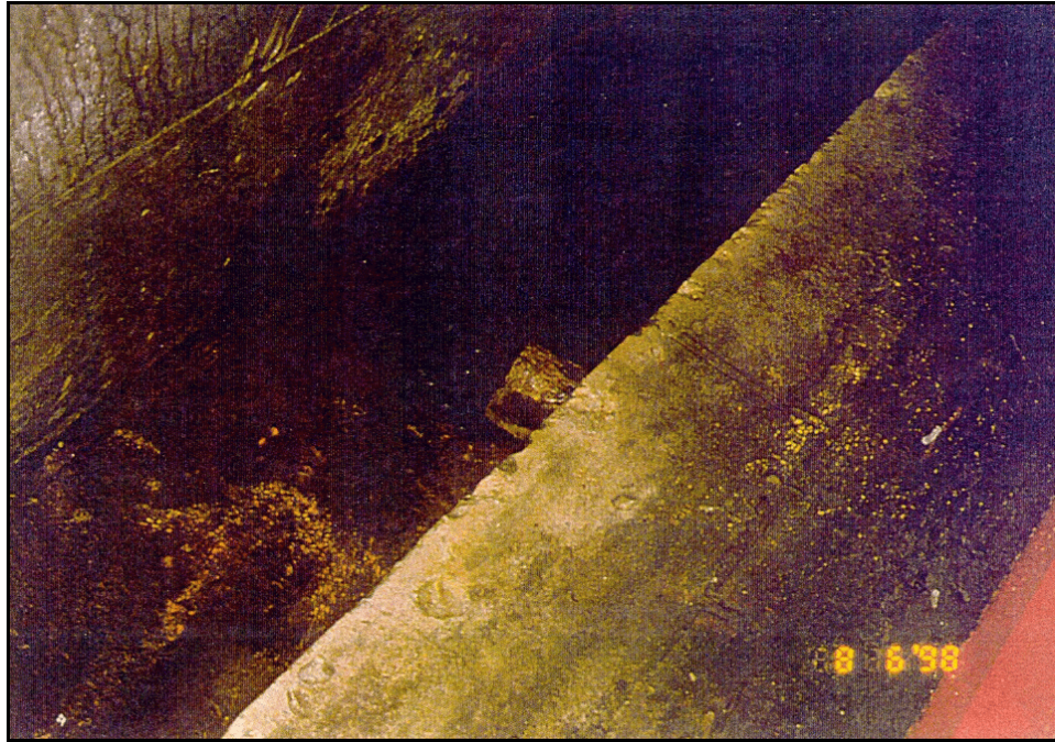
Figure 4. —Gutter along the upstream side of the foundation gallery. The outlet of a lateral discharge pipe is shown near the center of the photograph. It connects to a nearby drain. Most of these pipes were at least partially plugged prior to the drain cleaning operation.
