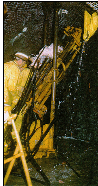
Figure 45. —Views of rotary drilling operations to install high-angle drain holes in bedrock in a drainage adit in the downstream right abutment of Horse Mesa Dam, Arizona. The drill rig is a Craelius Diamec 260. The drill is mounted on a stand when drilling high-angle drain holes.
