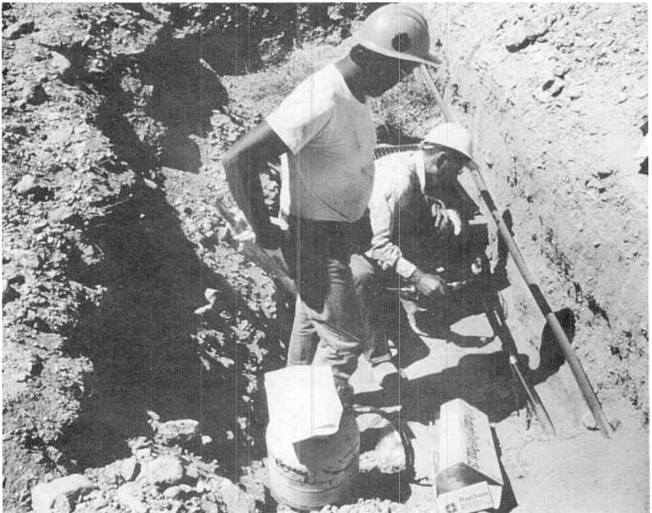
Figure 3-20. — Installation of buried cable.
