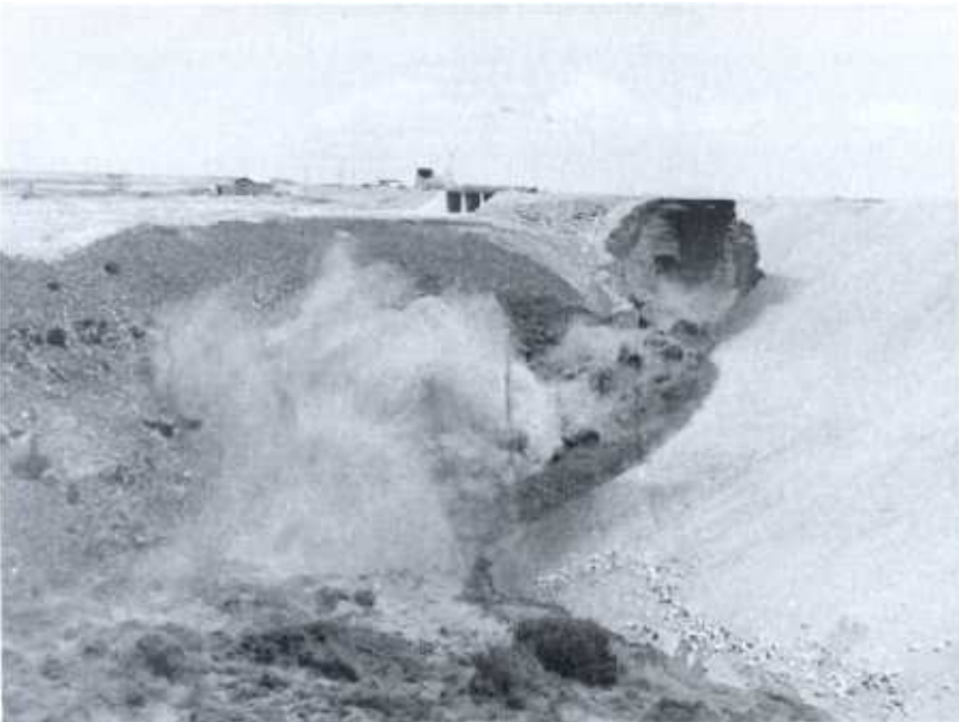
Figure 4-16.—Teton Dam failure sequence, June 5, 1976—Continued.
