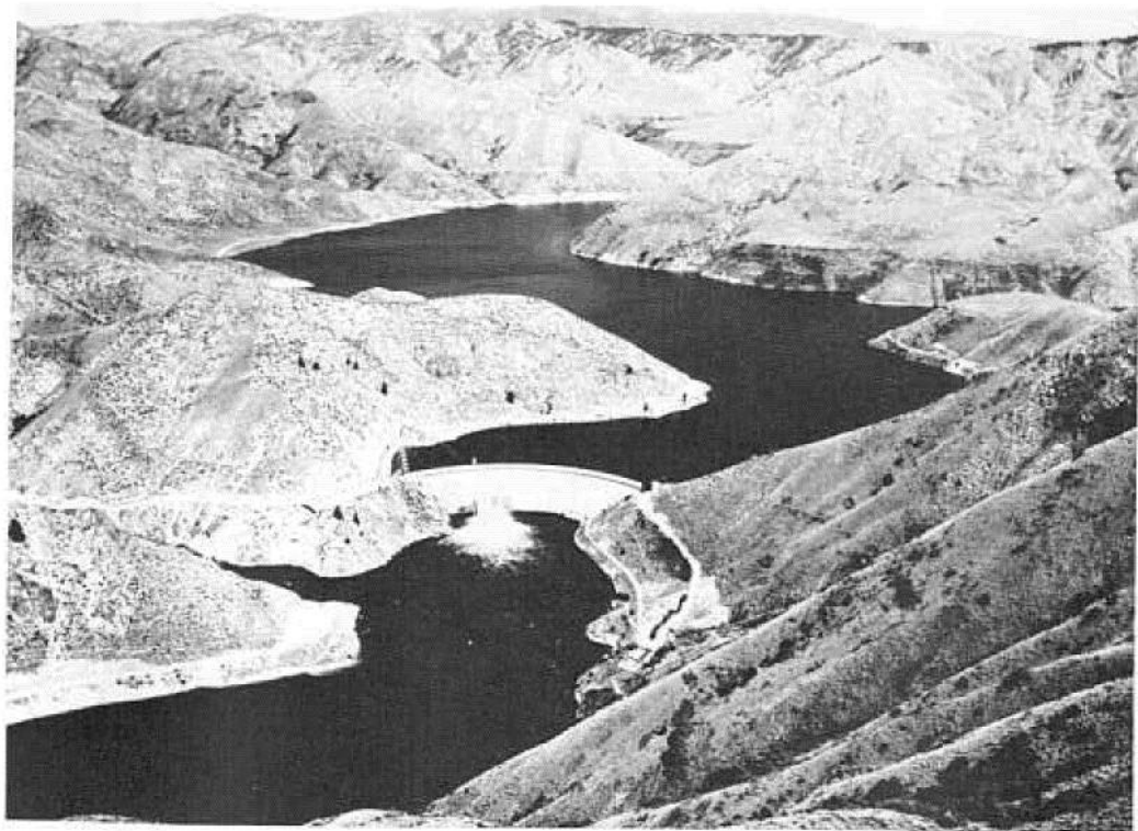
Figure 1-38.—Arrowrock Dam (P4-100-8511). P-801-D-79324.
