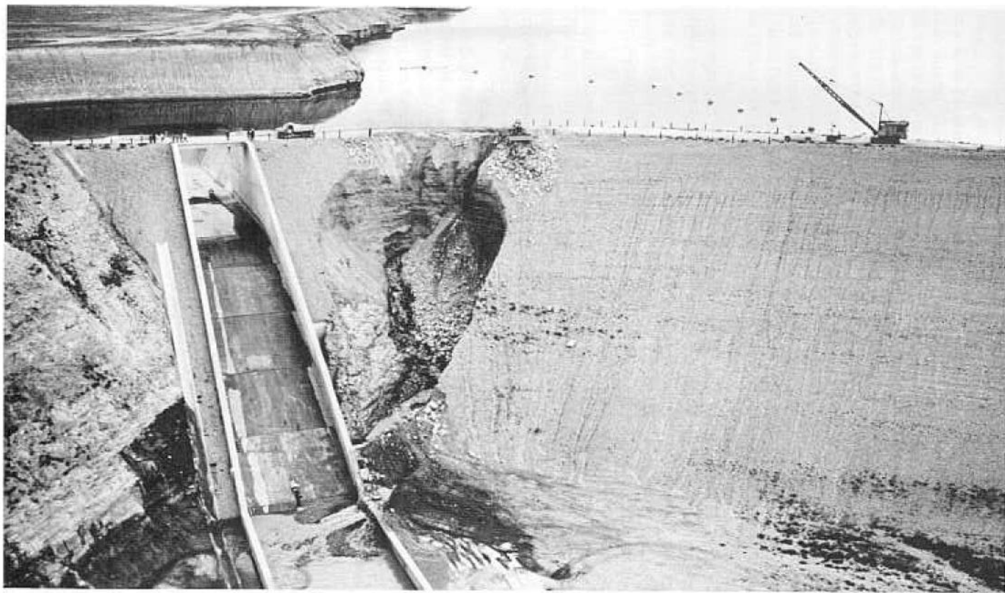
Figure 4-4.—Fontenelle Dam (P154-400-1501). P-801-D-79349.
