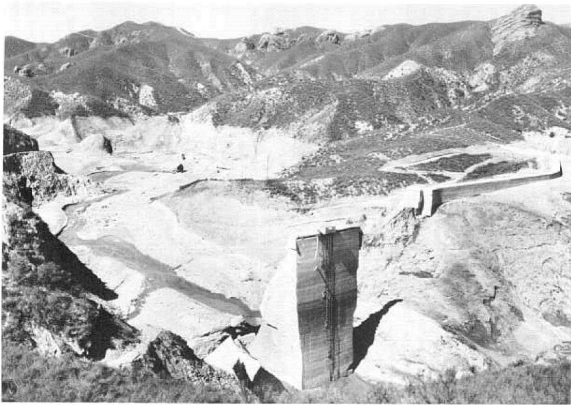
Figure 4-11.—St. Francis Dam after failure (Courtesy, Calif. Dept. of Water Resources). P-801-D-79356.
