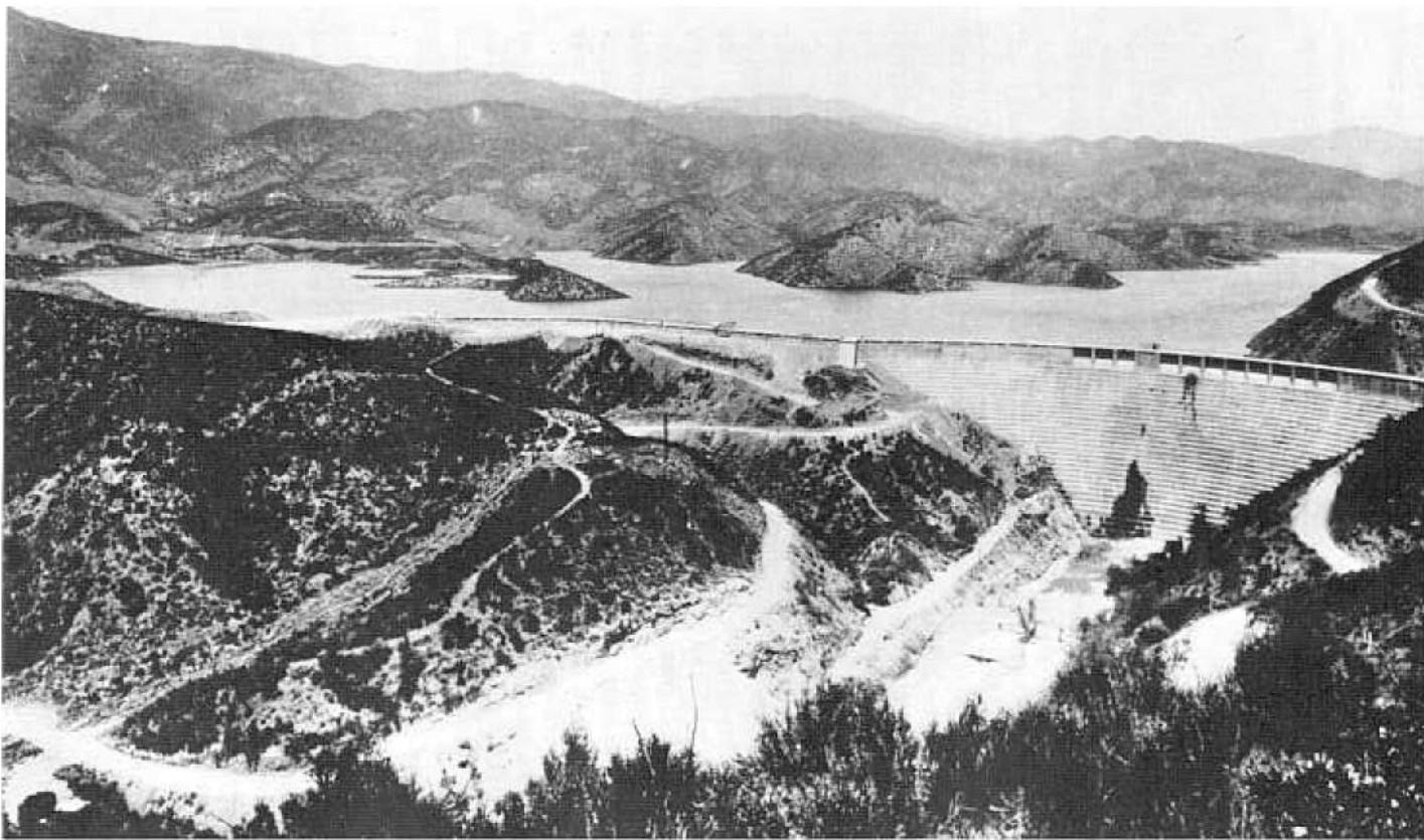
Figure 4-10.—St. Francis Dam before failure (Courtesy, Calif. Dept. of Water Resources). P-801-D-79355.
