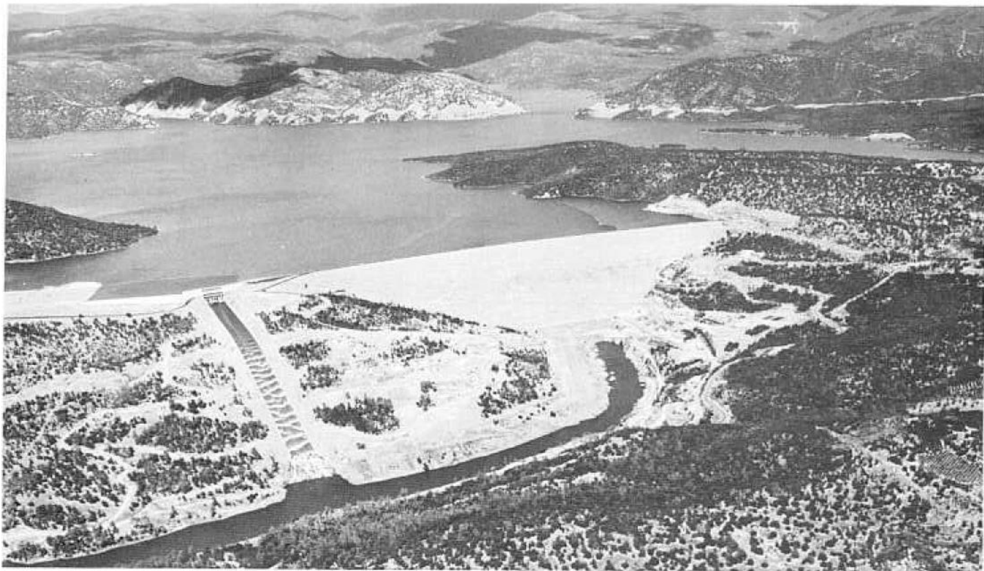
Figure 1-48.—Oroville Dam (Courtesy, Calif. Dept. of Water Resources), P-801-D-79334.
