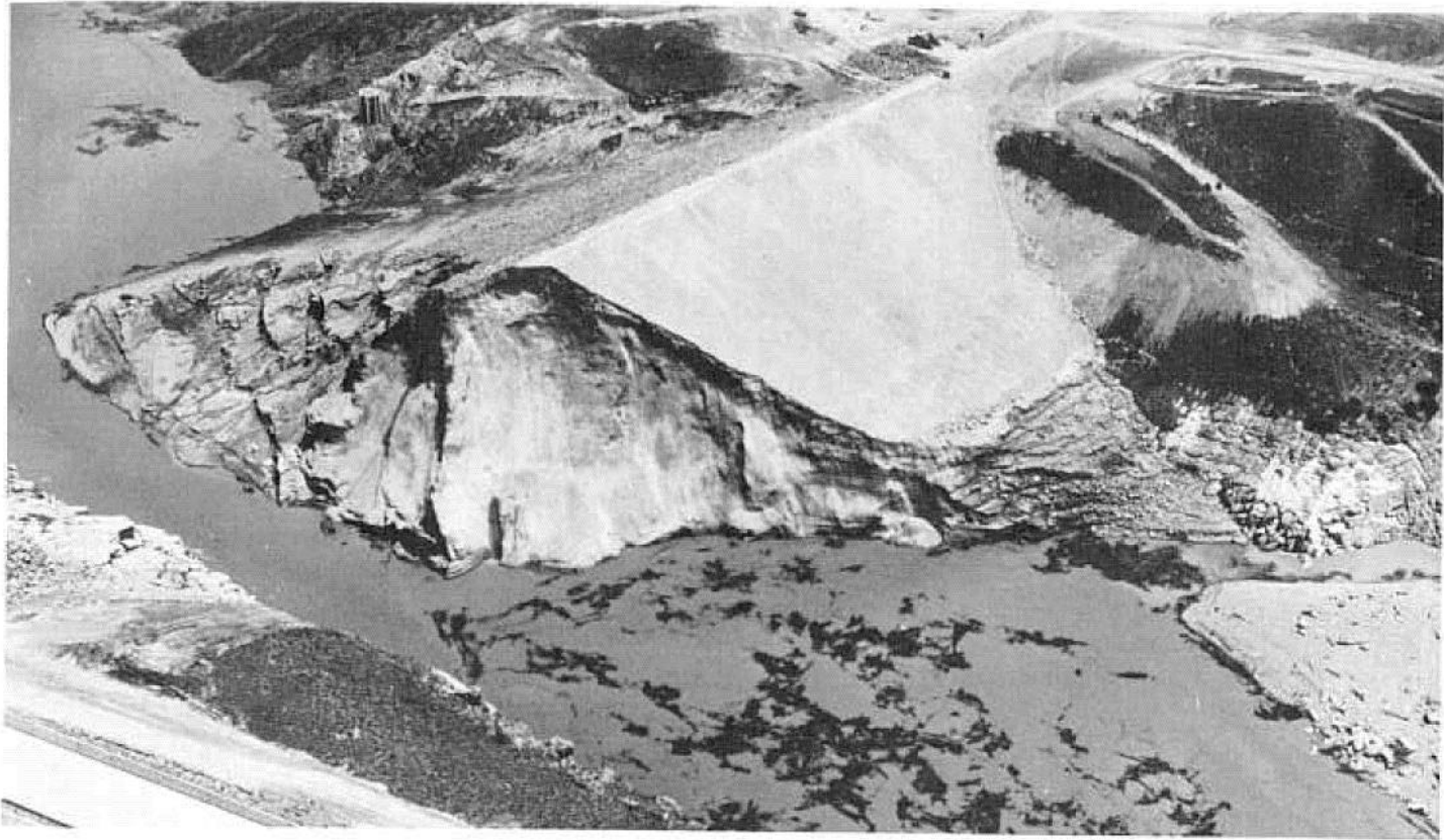
Figure 4-17.—Teton Dam, downstream view after failure (P549-100-215A). P-801-D-79368.
