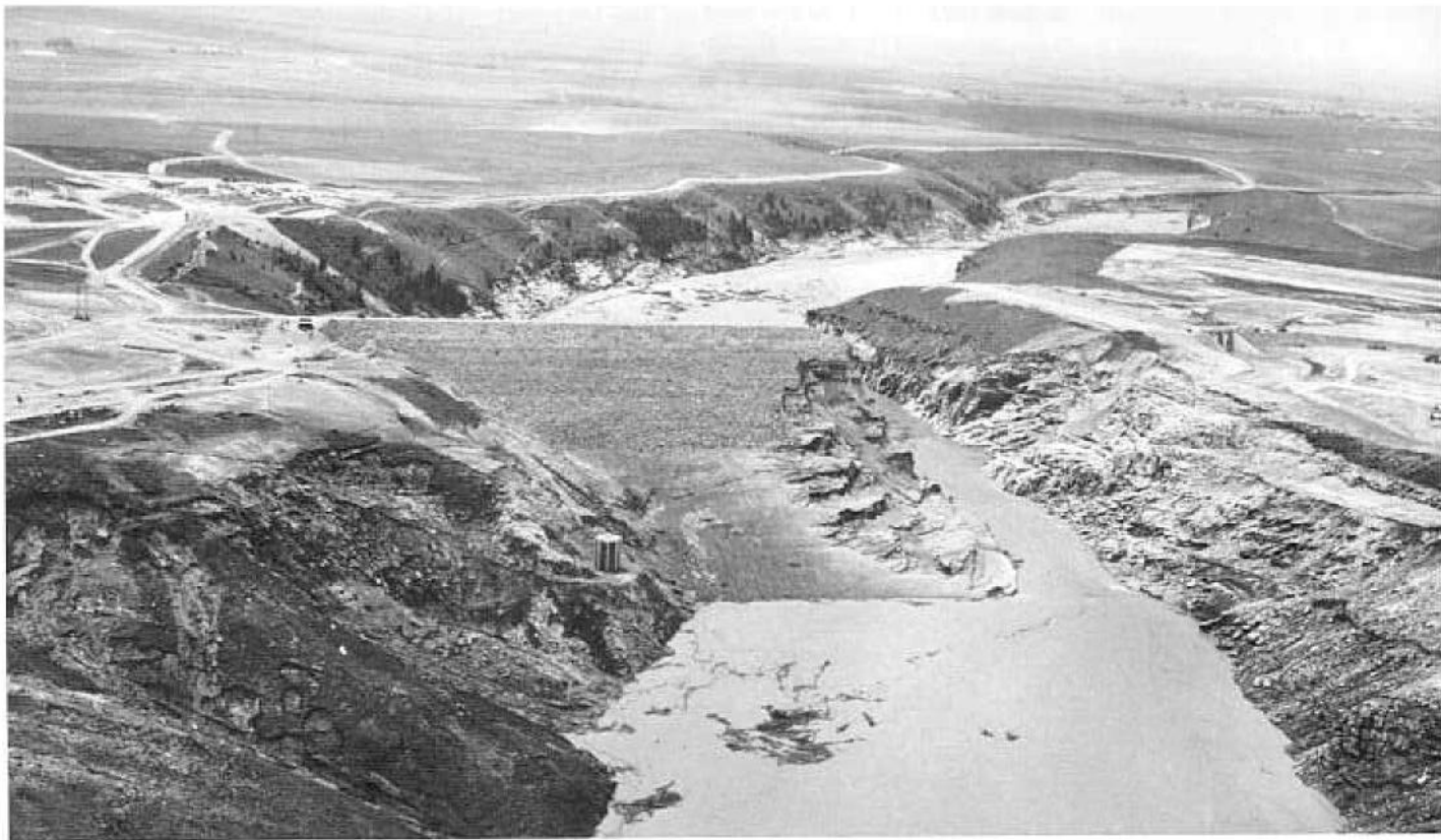
Figure 4-18.—Teton Dam, upstream view after failure (P549-100-218A). P-801-D-79369.
