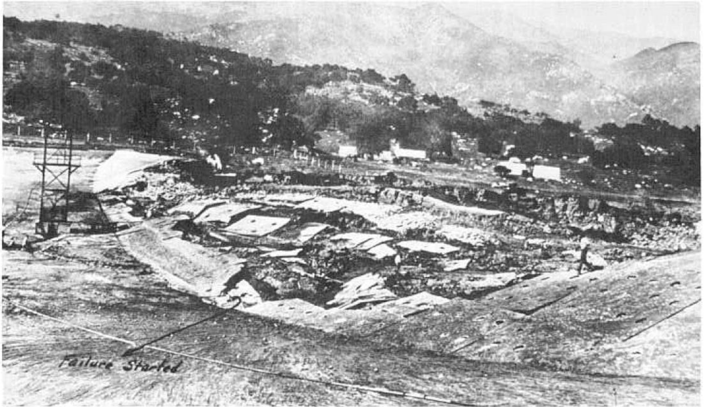
Figure 5-1.—Sheffield Dam following failure (Courtesy, Calif. Dept. of Water Resources. P-801-D-79382.
