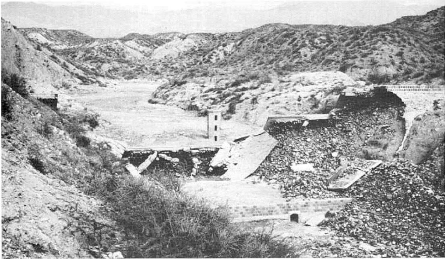
Figure 4-5.—Frías Dam after failure, downstream view (Courtesy of C. J. Cortright). P-801-D-79350.
