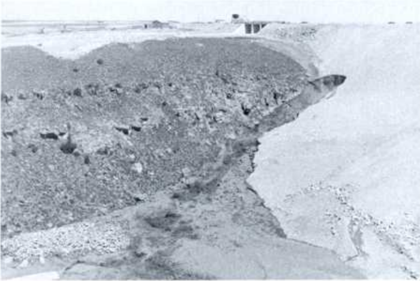
Dozers lost in hole, about 11:20 a.m. P-801-D-79364 (top).
