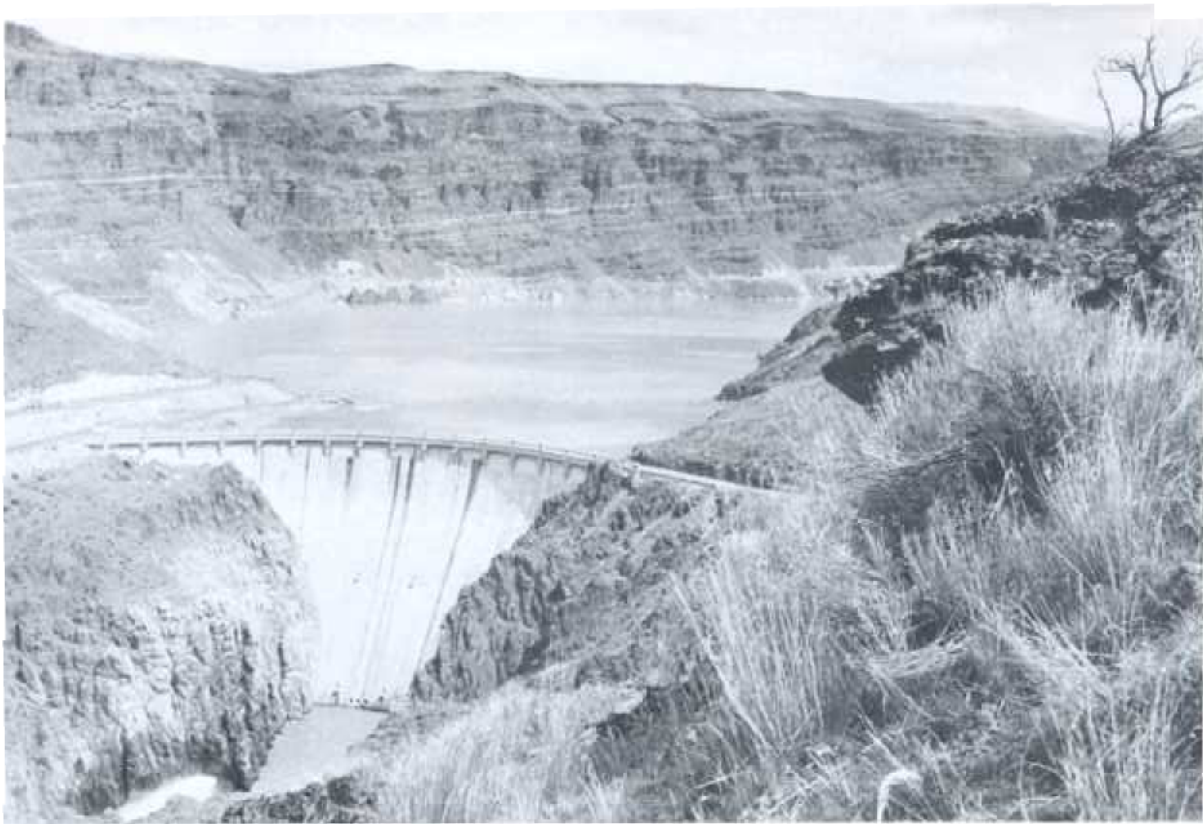
Figure 1-41.—Owyhee Dam (P48-100-413I). P-801-D-79327.
