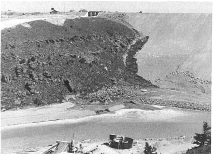
Figure 4-16.—Teton Dam failure sequence, June 5, 1976.
