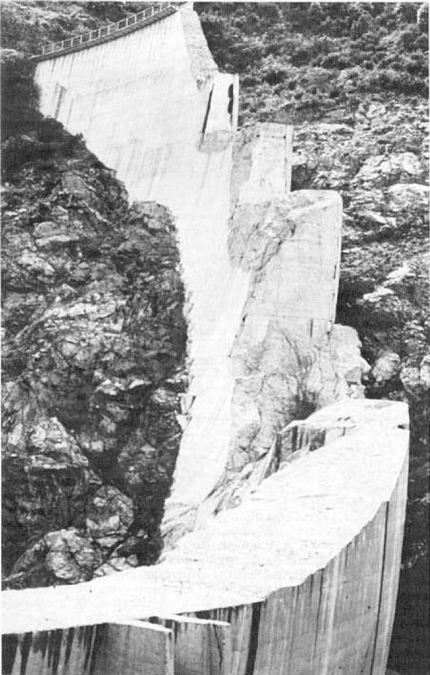
Figure 4-8.—Malpasset Dam, right abutment, showing remnant (Courtesy of L. B. James). P-801-D-79353.
