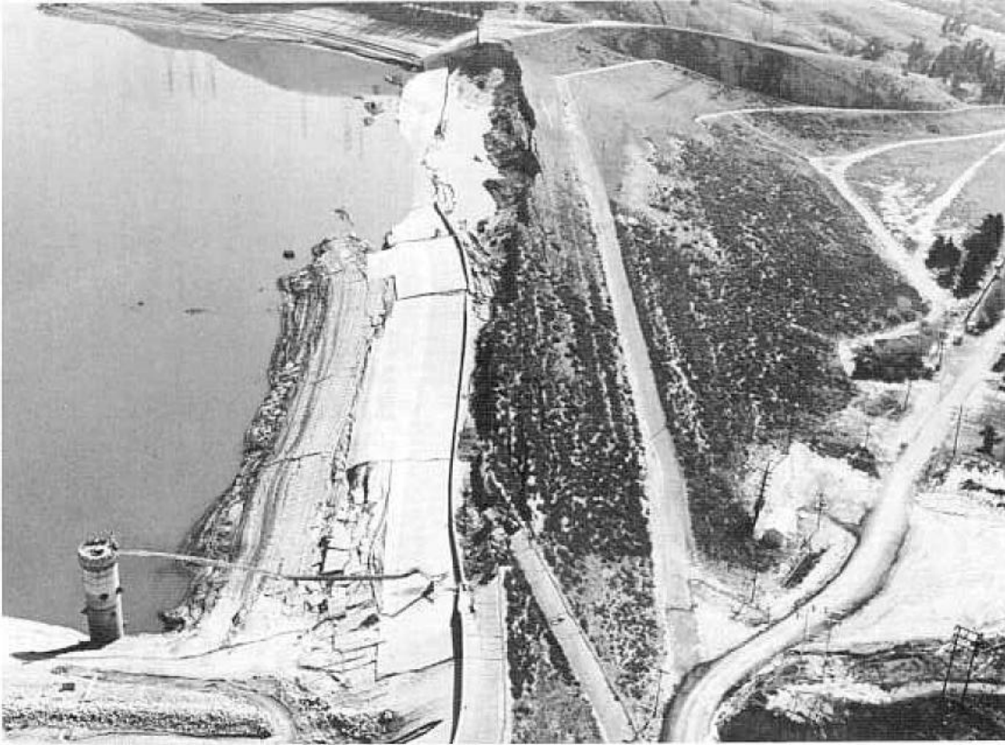
Figure 4-26.—Lower Van Norman (San Fernando) Dam after earthquake of February 9, 1971 (Courtesy, Calif. Dept. of Water Resources). P-801-D-79378.
