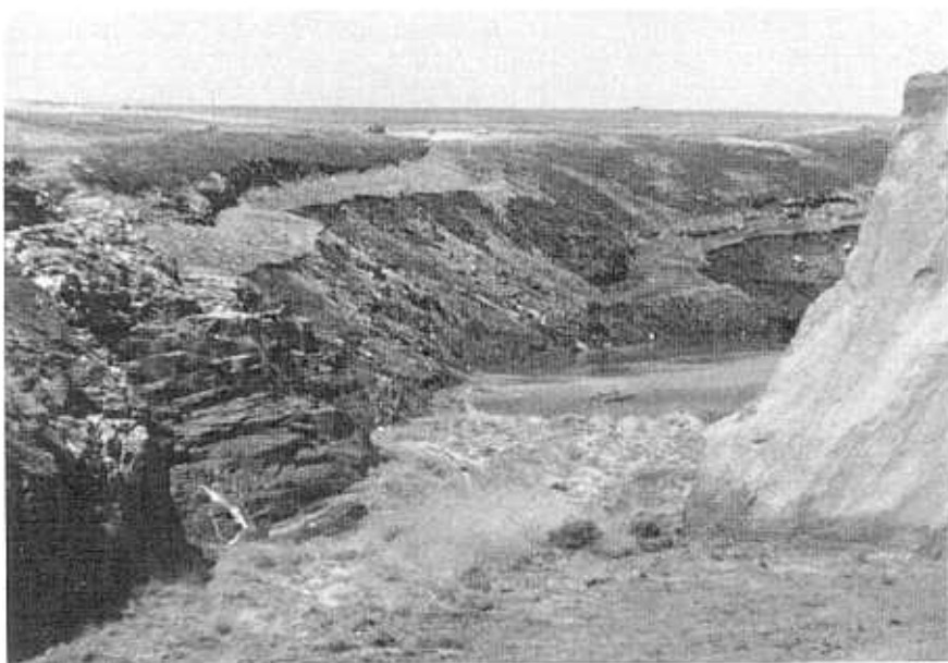
Figure 4-16.—Teton Dam failure sequence, June 5, 1976—Continued.
