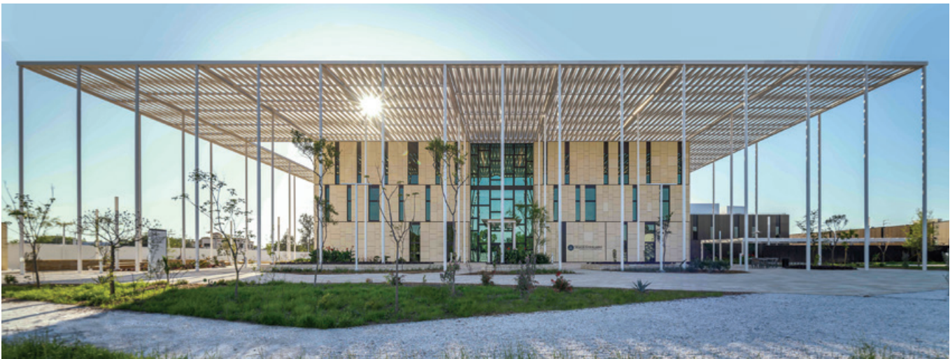
The new U.S. Consulate General Matamoros, Mexico is situated on a 7.6-acre compound. The project was dedicated in May 2019.
