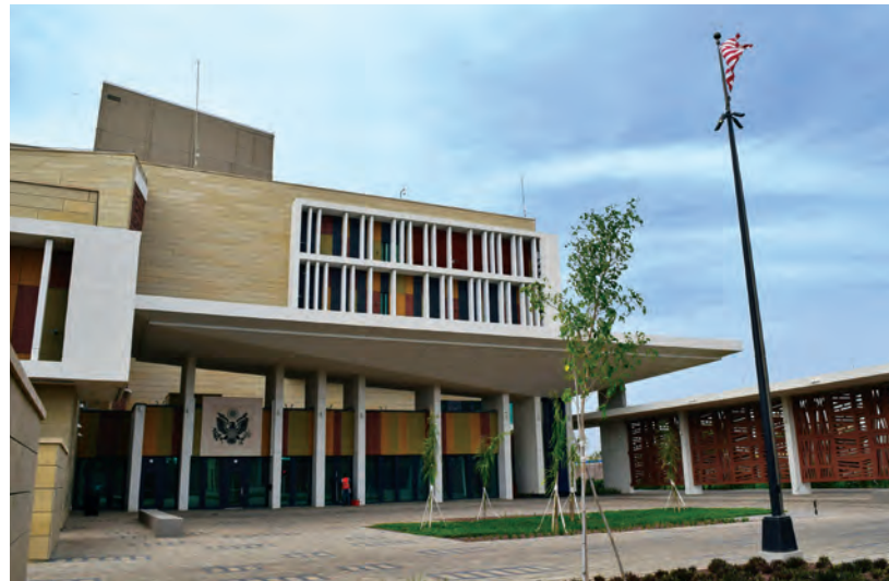
The new U.S. Embassy in N'Djamena, Chad, situated on a 12-acre site, includes supporting buildings for the Chancery, Marine Security Guard, and the Embassy community. Department of State/OBO
