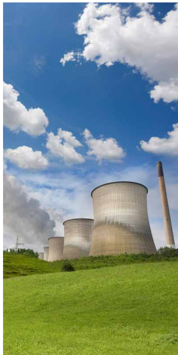
A cooling tower is a heat exchanger that cools water that was used to cool exhaust steam from a power plant's turbines ( Definition source: nrc.gov ).
