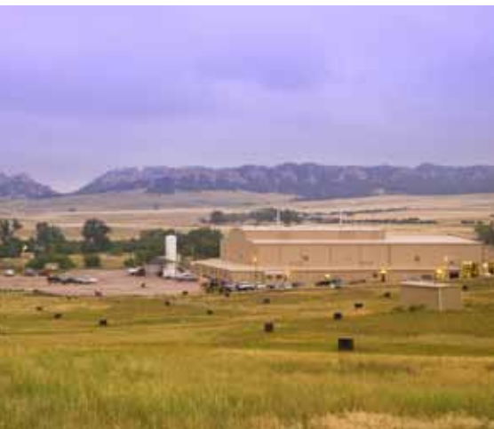
The Cameco Corporation Crow Butte uranium mine in northeast Nebraska.
