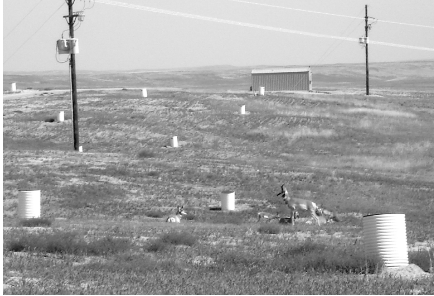
Figure 3-4. Wellheads and Header House, Smith Ranch, Converse County, Wyoming (NRC 2009, Figure 2.1-4)
