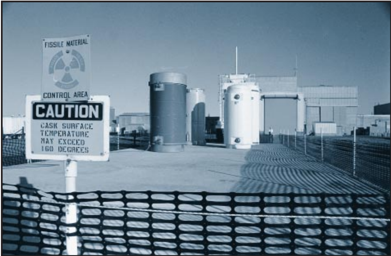
Providing dry aboveground storage for spent fuel in special casks is one possible alternative to underwater storage. Spent Fuel Storage-Cask Testing Pad, Test Area North, Idaho National Engineering Laboratory. March 17, 1994.
