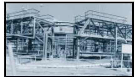
5. To make space for more liquid high-level radioactive waste in the storage tanks, we built evaporators to reduce the waste volume.
