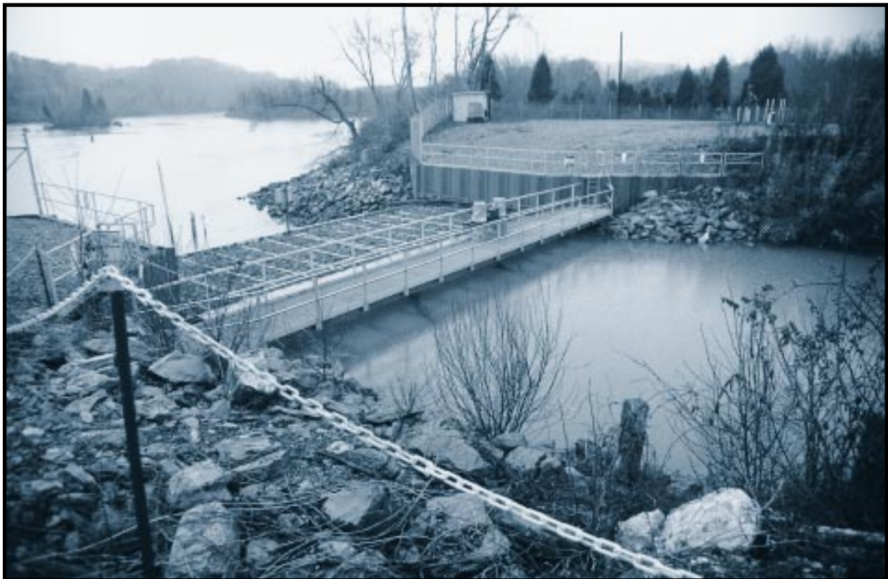
The White Oak Creek embayment is sited where the Clinch River meets White Oak Creek, whose waters flow through the site of the Oak Ridge National Laboratory. When creek waters leave the site, they are contaminated with cesium 137, strontium 90, and PCBs. Until 1991 there was a cable with a warning sign at this point. In 1992 the Department constructed a state-of-the-art sediment-retention dam that uses interlocking sheets of metal driven into bedrock to retard the flow of water so that contaminated sediments can settle behind the dam. Oak Ridge, Tennessee. January 11, 1994.
