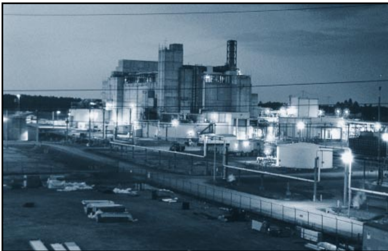
This vitrification plant for high-level waste is 120 yards long and encompasses 5 million cubic feet. It contains 69,000 cubic yards of concrete with 13,000 tons of reinforcing steel and 320,000 feet of electrical cable. It is designed to turn high-level waste into glass logs by pouring a mixture of waste and borosilicate glass into stainless-steel canisters, which are then sealed and stored. Workers completed major testing in 1995, including producing more than 70 canisters of test glass. Defense Waste Processing Facility, Savannah River Site, South Carolina. January 7, 1994.
