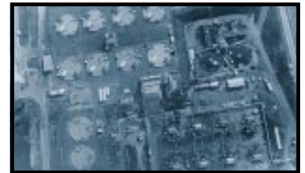
3. To store the liquid high-level radioactive waste from the reprocessing canyons, we built underground storage tanks.
