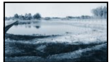
6. To dispose of wastewater that the evaporators removed from the high-level waste tanks, we built seepage basins.
