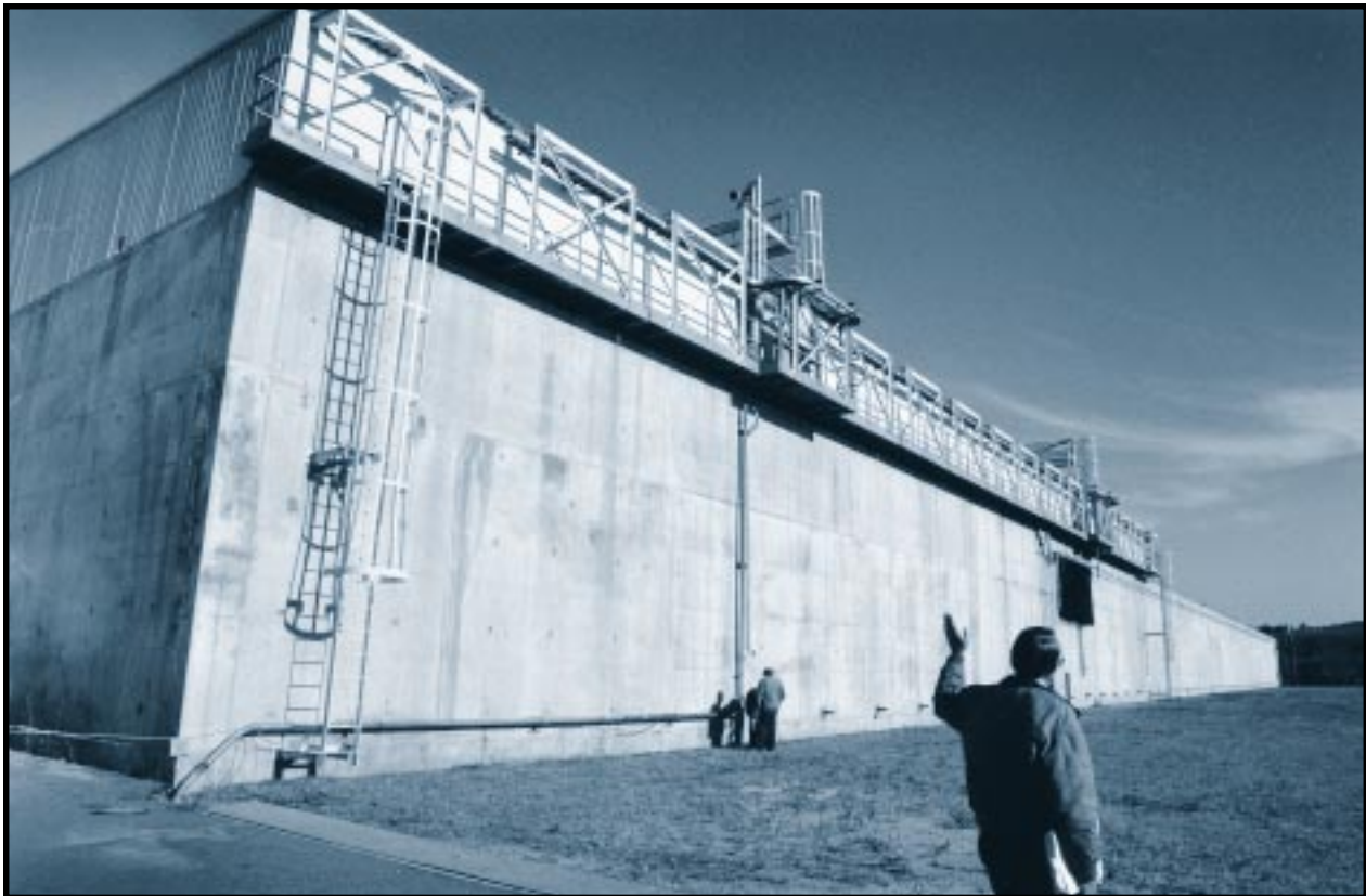
The Z-Area vault for low-level-waste in saltstone form is a 25-foot-tall reinforced-concrete structure 600 feet long and 200 feet wide, housing 12 concrete cells that will be filled with solid grout. The grout is made of a low-level radioactive solution mixed with cement, fly ash, and slag. The chief radionuclides locked into the grout are technetium 99, strontium 90, and cesium 137. Once all 12 cells are filled, the vault will be covered with earth and capped with clay. Savannah River Site, South Carolina.
