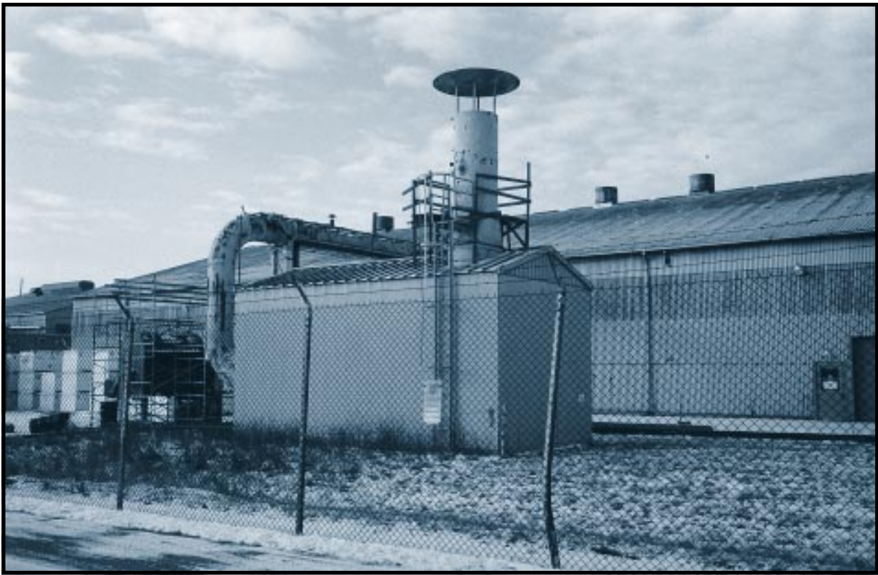
This exhaust stack was used to control emissions from the Plant 9 facility, where enriched uranium materials were processed. The malfunctioning of systems like this resulted in several releases of uranium dust, totalling several hundred tons, to the environment outside the plant buildings over the course of operations. Fernald Plant, Ohio. December 30, 1993.
