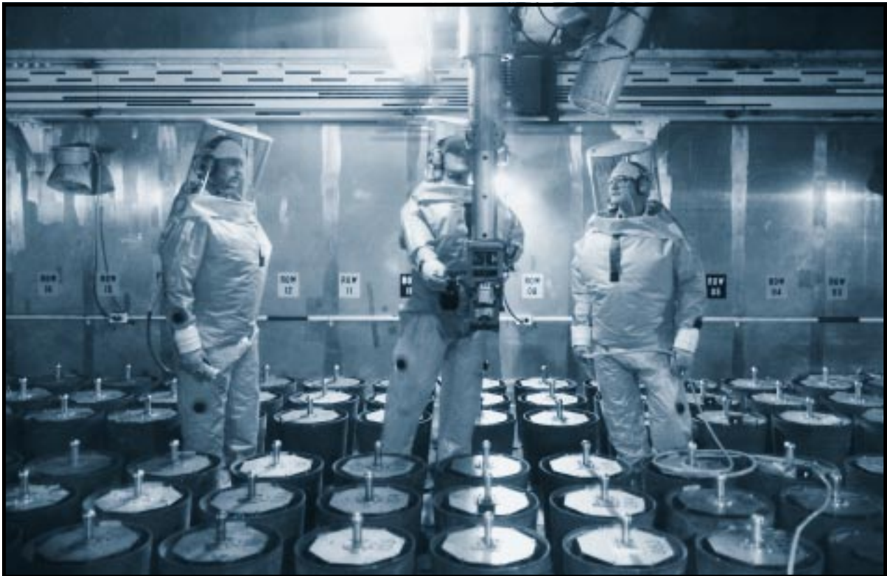
The X-Y Retriever Room at the Rocky Flats Plant contains plutonium in many forms. During normal operations, plutonium in this room was recycled for warhead production. Today the room is used to store surplus plutonium. Here workers are making repairs to a hoisting mechanism. The hoist is used to lift the plutonium from the storage cans on the floor. Building 707, Rocky Flats Plant, Colorado. November 29, 1988.
