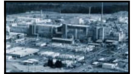
2. To extract plutonium from reactor targets, we built reprocessing "canyons," which generated liquid high-level radioactive waste.
