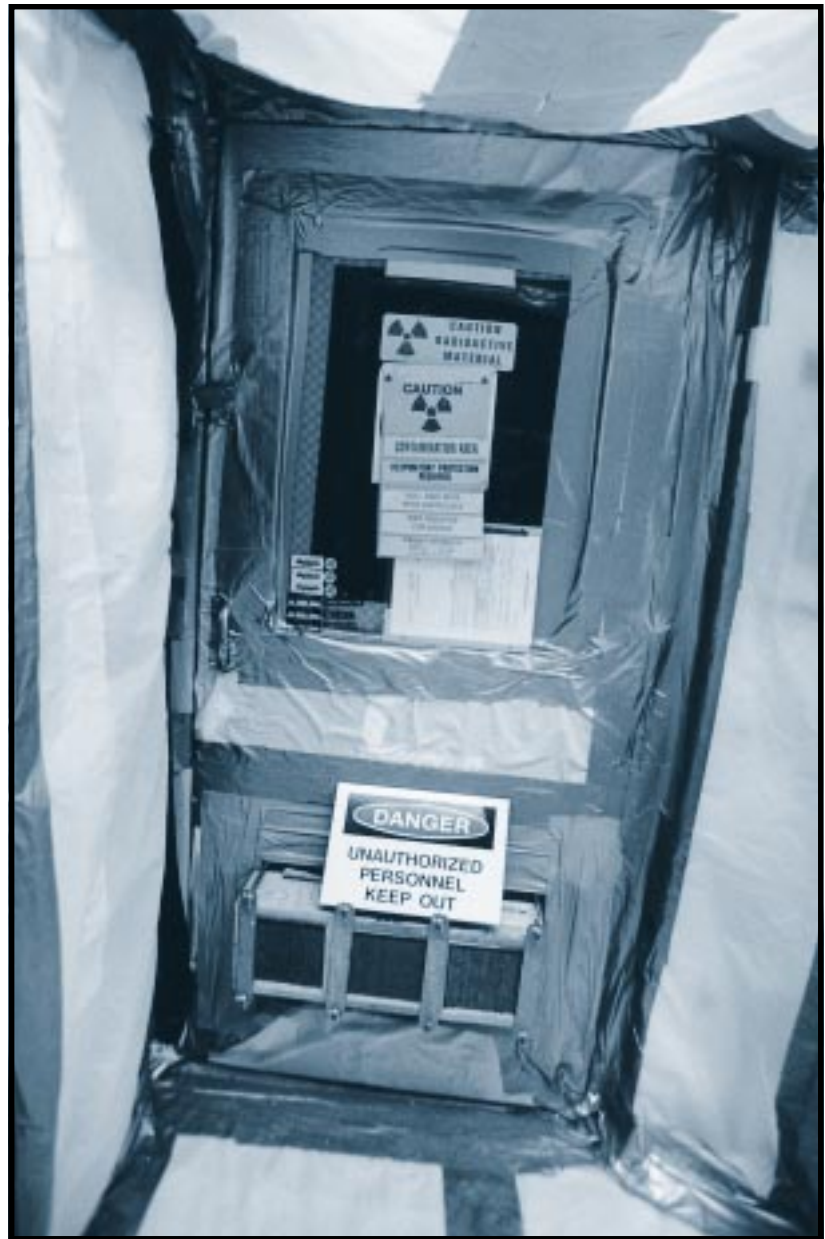
The sealed door to an “infinity room” at Rocky Flats. More than 20 such rooms have been contaminated by releases during plutonium operations at the site. The rooms are called “infinity rooms” because the rates of alpha radiation are too high for standard monitoring equipment to measure. The radioactivity in these rooms is nearly 25,000 times natural background. Building 776/777, Rocky Flats Plant, Colorado. March 18, 1994.
