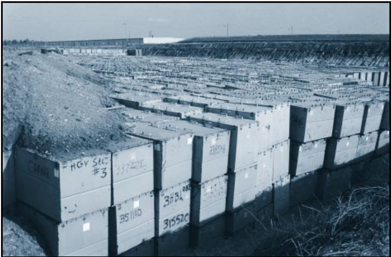
This engineered trench for low-level waste contains approximately 30,000 stacked carbon-steel boxes of waste, each box being 4 by 4 by 6 feet. It stopped receiving waste in 1995. In 1996, the site will be backfilled with dirt to form a mound, which will be seeded with grasses and sloped for runoff. Once this trench is closed, the trench-burial of low-level waste here will stop. Engineered Low Level Trench 4, Solid Waste Management Burial Grounds, Savannah River Site, South Carolina. January 7, 1994.
