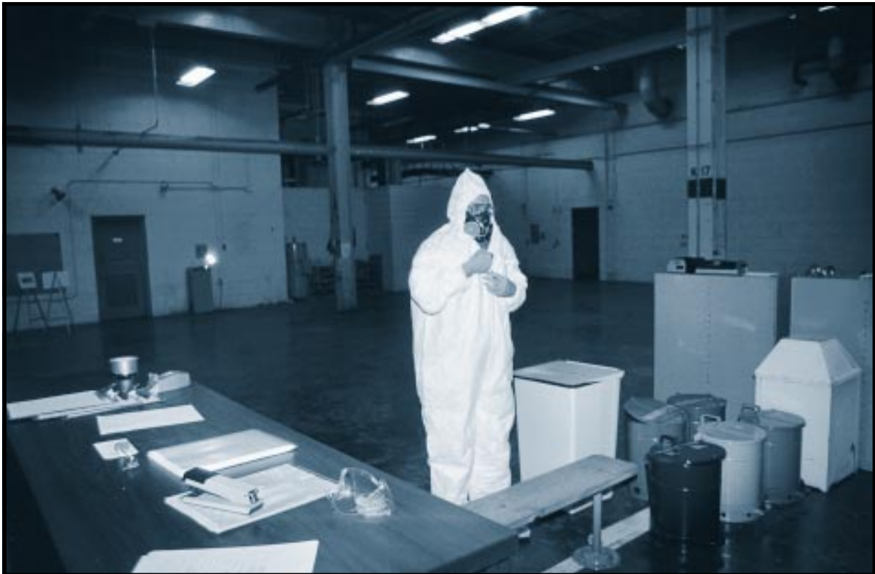
During the cleanup of mercury contamination, this worker uses a special suit and respirator for protection against mercury-vapor poisoning. Many tons of mercury were released to the environment at Oak Ridge's Y-12 Plant during lithium-enrichment operations. Enriched-lithium targets are needed to make tritium, a radioactive gas used in nuclear weapons. Oak Ridge, Tennessee. January 11, 1994.
