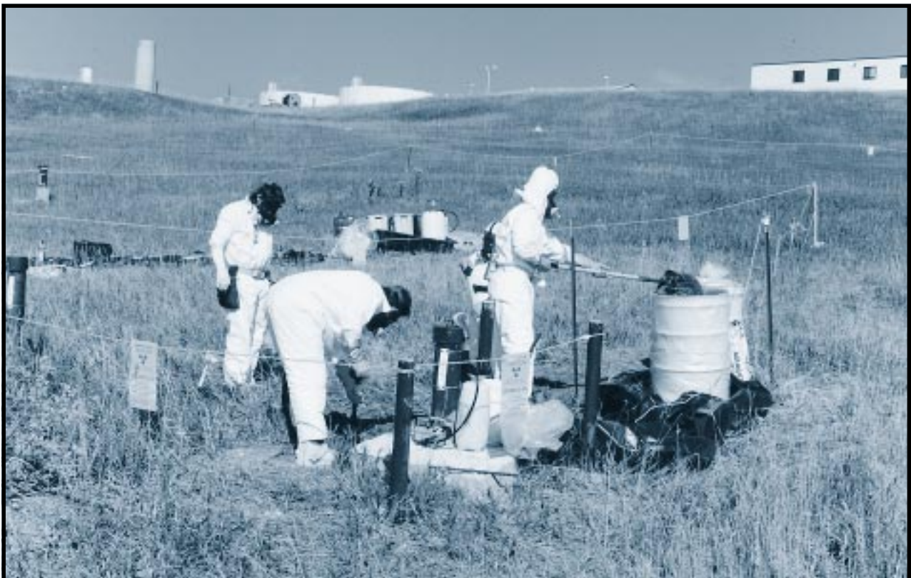
Workers remediate the 881 Hillside at Rocky Flats, an area that became heavily contaminated with toxic and radioactive substances. As part of the remediation action at the site, workers cleaned up six “hot spots” of highly radioactive contaminated soil. Rocky Flats Plant, Colorado. September 1994.
