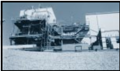
10. To reduce the volume of liquid high-level waste, we built the In-Tank Precipitation Facility.
