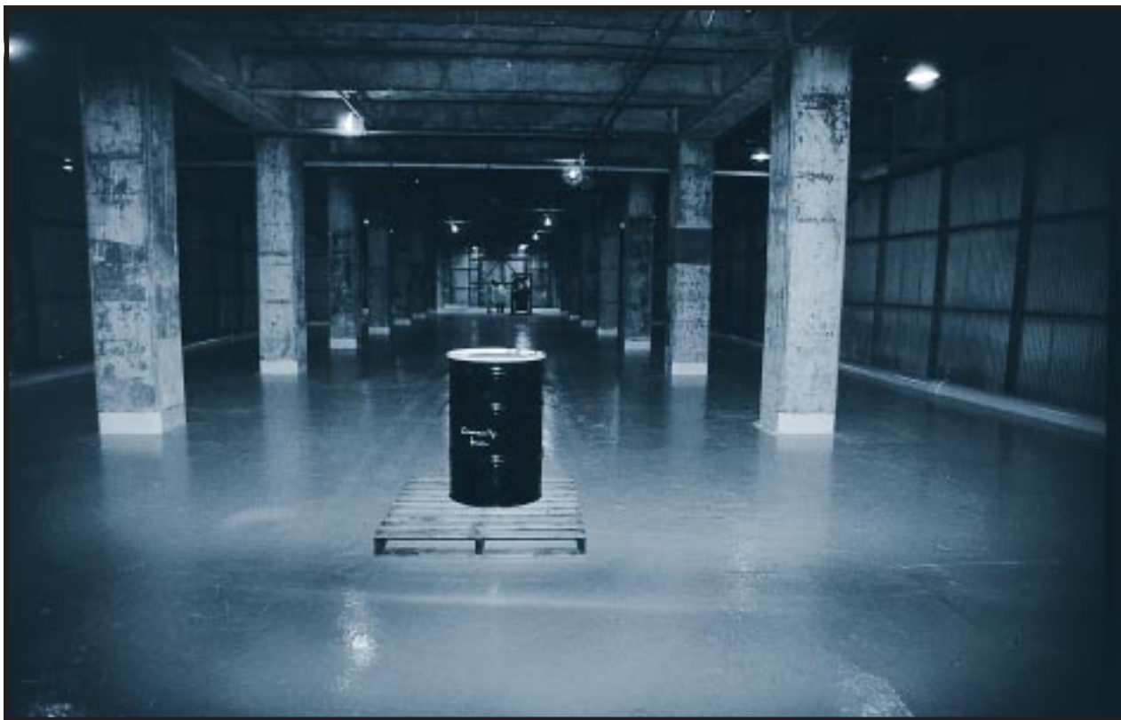
A 55-gallon drum ready for storage in the basement level of the K-25 Gaseous Diffusion Plant. K-25 has prepared 45 basement vaults for the storage of low-level and mixed hazardous wastes. These vaults will be able to hold some 63,000 drums. A coat of epoxy sealant covers the renovated vault floor, adding one more level of containment for wastes stored here. K-25 Gaseous Diffusion Plant, Oak Ridge, Tennessee. January 10, 1994.
