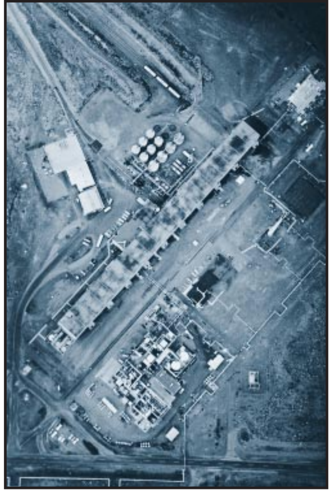
The B Plant canyon was the world's second large-scale reprocessing facility. It dissolved irradiated fuel rods in acid to recover plutonium. Hanford Site, Washington. November 15, 1984.
