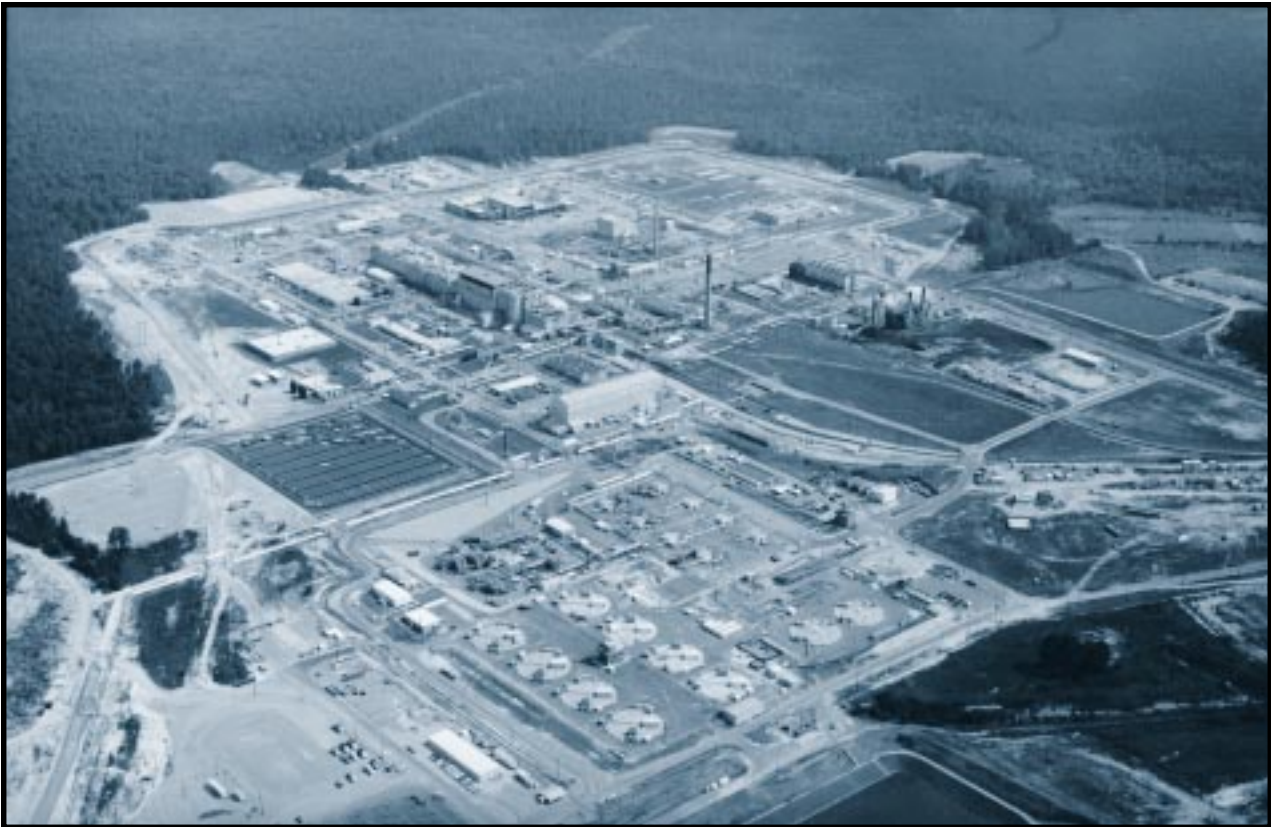
Aerial view of the F Area at the Savannah River Site. This is one of the two chemical separation areas at the site. It covers just over half a square mile. All facilities shown on the facing page are within 5 miles of this spot. Visible in this photograph are the F Area Seepage Basin before closure (lower right), the F Area Tank Farm (group of circles near the bottom center), the 242-F Evaporator (between the two rows of tank tops), and the 221-F Canyon (long building above parking lot). F Area, Savannah River Site, South Carolina. August 6, 1983.
