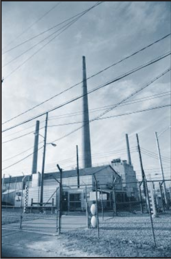
This tritium facility extracted tritium gas from lithium reactor targets. Savannah River Site, South Carolina. January 7, 1994.
