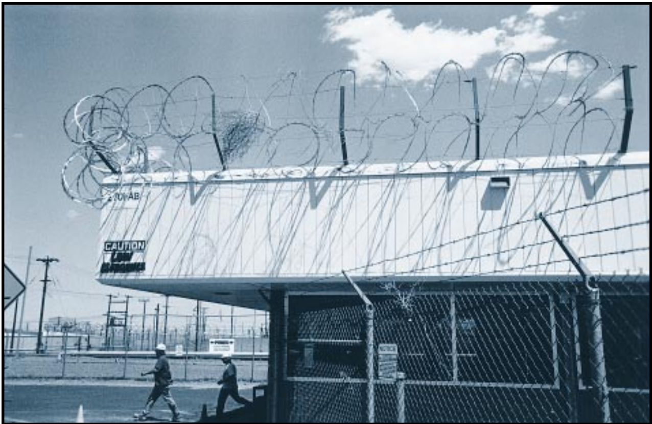
This high-security fence at Hanford's Plutonium-Uranium Extraction (PUREX) Plant was designed to safeguard strategic nuclear materials. Currently, this guardhouse, once staffed with guards, is used as an entry point for employees. PUREX operations ceased in 1990. Hanford Site, Washington State. July 11, 1994.
