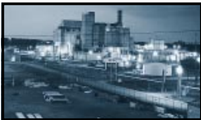
9. To stabilize the liquid high-level radioactive waste in the storage tanks, we built the Defense Waste Processing Facility.
