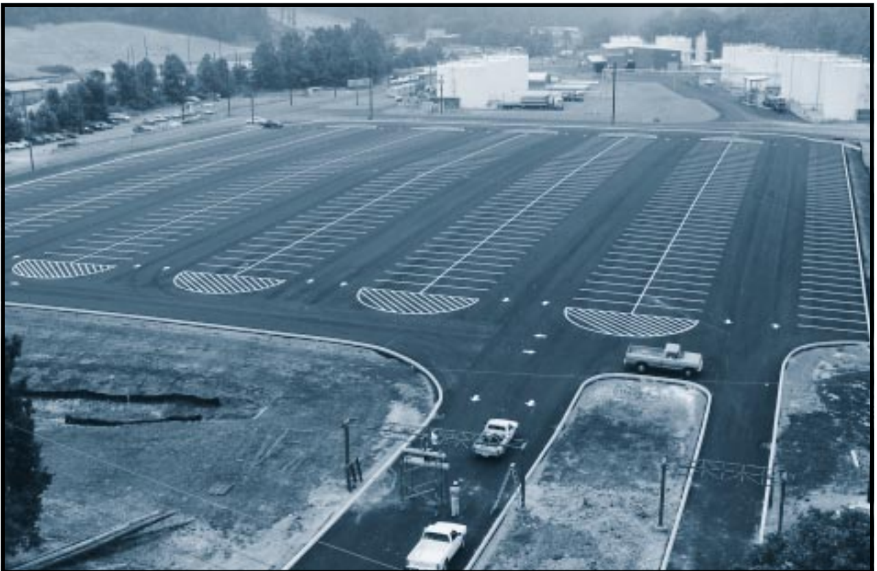
AFTER – A parking lot is now located where the four ponds shown above once stood. The liquids in these ponds were treated to remove contaminants beginning in 1985; the ponds were then drained and capped with asphalt. The project was completed in 1990. Oak Ridge, Tennessee.
