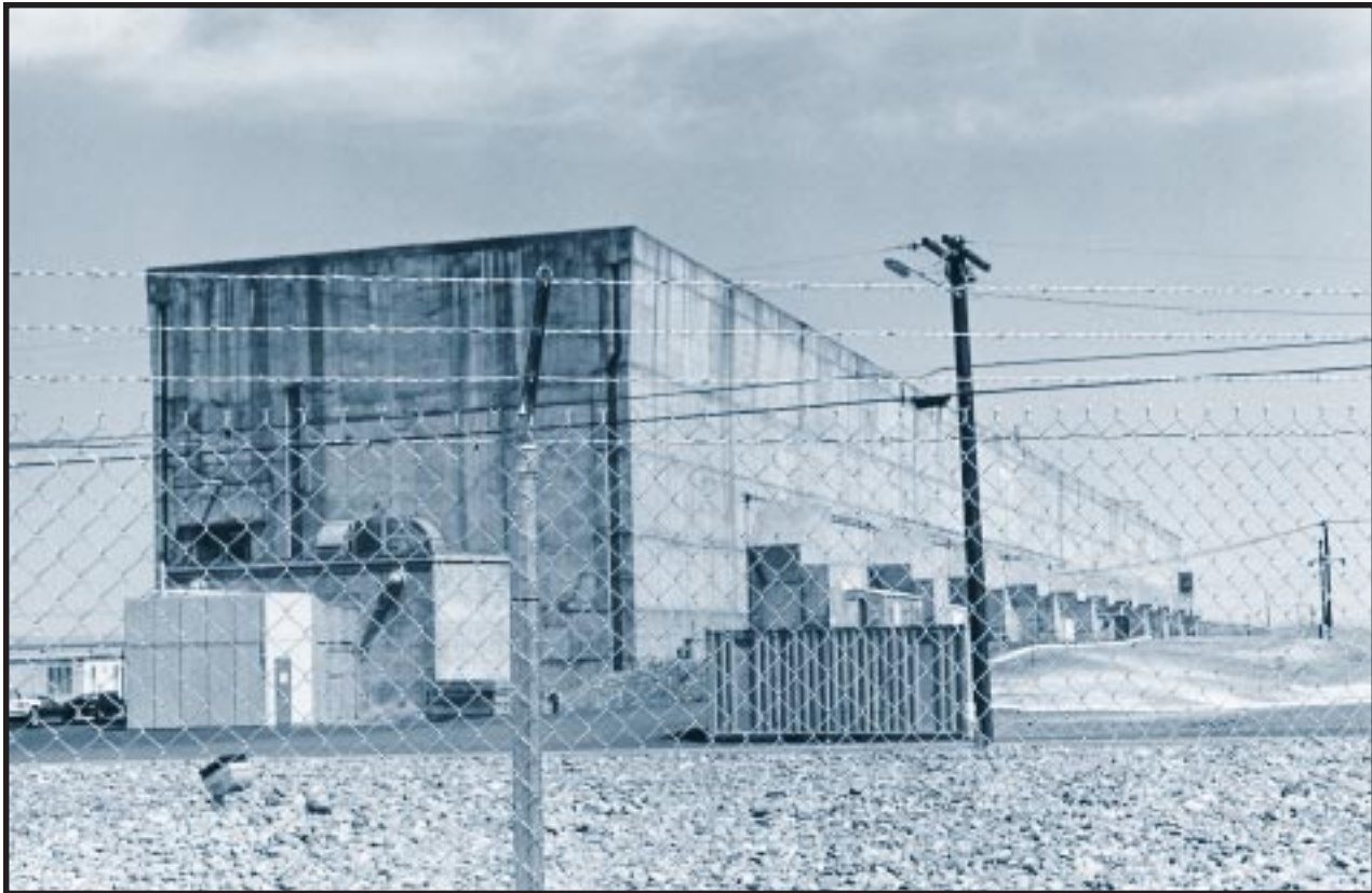
The T Plant was the world's first reprocessing canyon. In 1944, it dissolved spent fuel from the Hanford B Reactor and chemically extracted the plutonium, which was then used to form the core of the Trinity and Nagasaki bombs. It continued reprocessing until 1956. Today, the plant is used to decontaminate equipment. Hanford Site, Washington. July 11, 1994.
