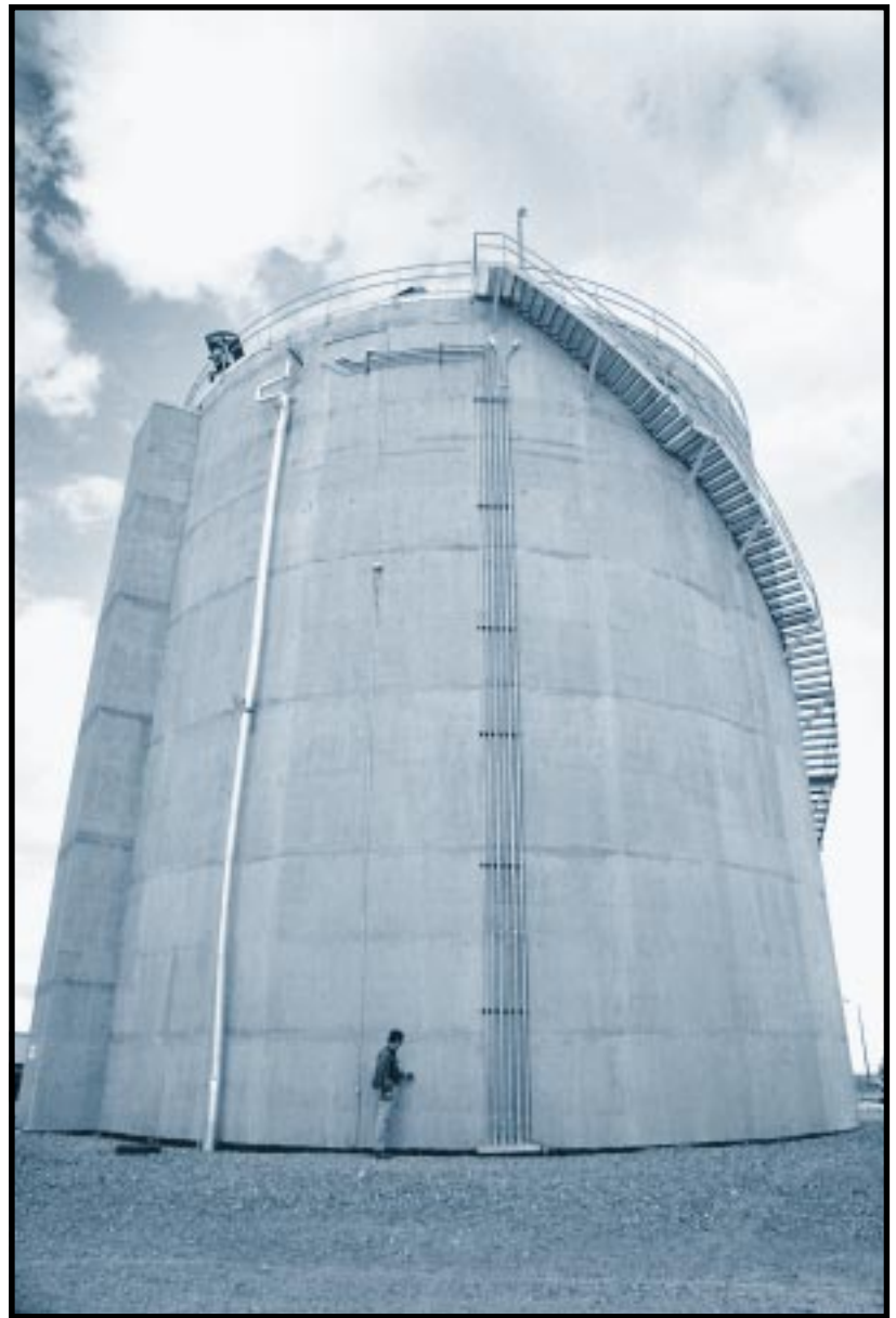
This storage bin for calcined high-level waste is made of reinforced concrete and steel. Inside its 4-foot-thick walls are stainless-steel silos containing up to 55,000 cubic feet of high-level waste in powdered form. There are seven bins like this in Idaho, and they are engineered to provide safe storage for 500 years. Idaho National Engineering Laboratory. March 17, 1994.
