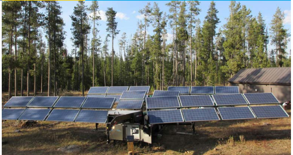
Figure 1. Mobile 9 kW Photovoltaic System at Bechler Meadows Ranger Station, Yellowstone National Park. Photo from DOE Federal Energy Management Program (FEMP)
