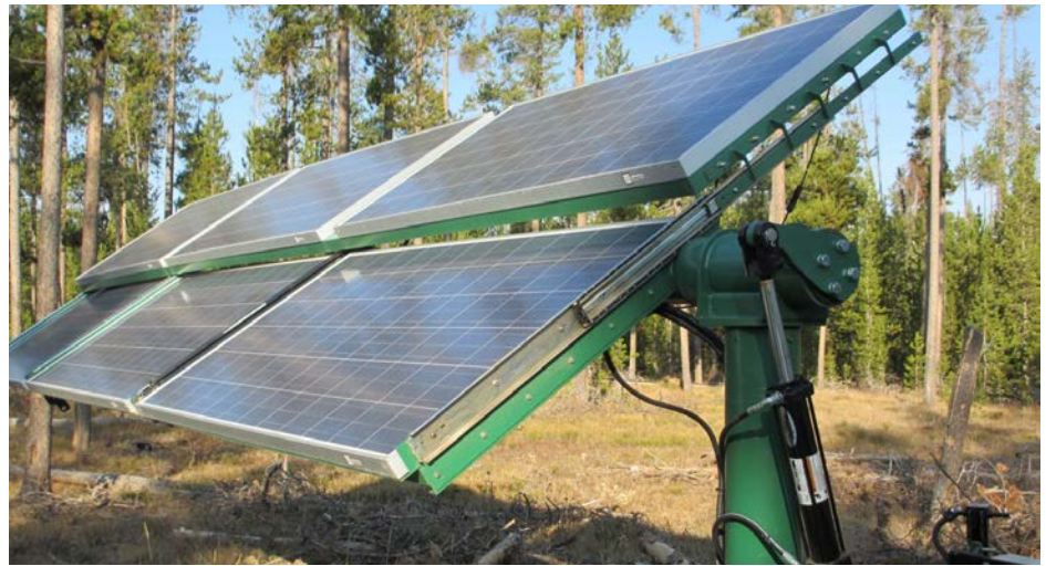
Figure 3. Hydraulic actuators rotate, unfold, and position the solar arrays. Photo: Andy Walker
