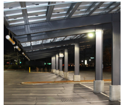
Figure 3. A parking lot recently retrofitted with covered parking. The covering incorporates PV panels that supply renewable energy to the site. Luminaires are mounted to the support structure for the PV panels.
