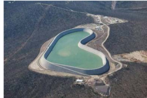
Pumped Hydro (Taum Sauk) 400 MW
