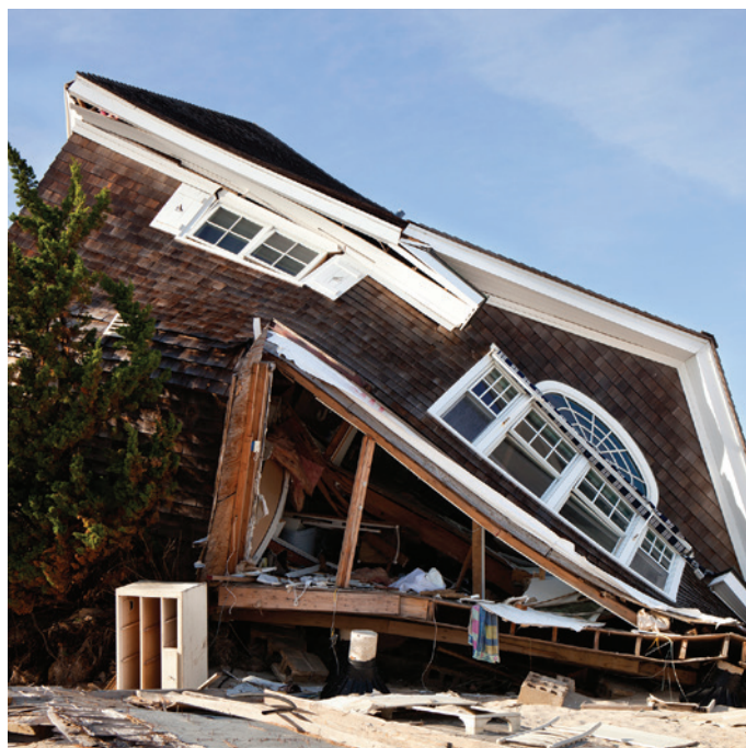
Storm-damaged home after Hurricane Sandy.
