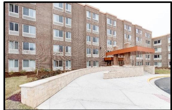
Tysons Towers in Vienna, VA, used RAD both to extend the property's affordability for another 20 years and to finance significant repairs to improve the quality of the housing for residents.
