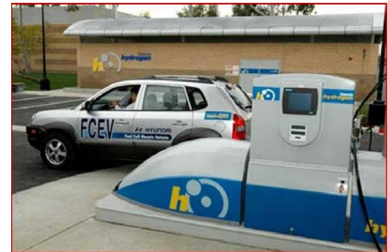
Chino, California Hydrogen Fueling Station
