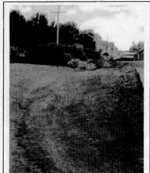
Figure 4. Site Drainage - The swale on the uphill side of the lot diverts water around to the side of the house.
