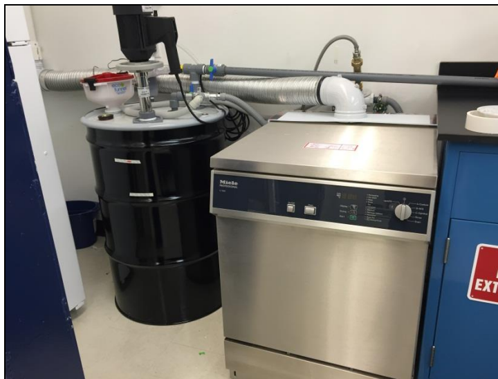
Figure 46. Miele G7899 washer-disinfector with wastewater decontamination system.
