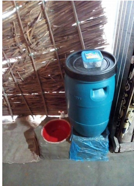
Drum with tap, installed inside the kitchen along with plastic bowl for basin
