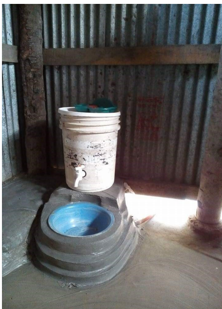
Used paint container with tap and installed inside the kitchen along with plastic bowl for basin
