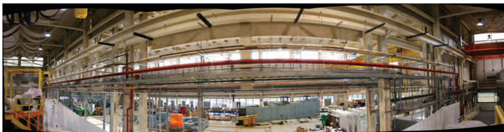
A distorted composite view of the new guide hall, looking through the removed columns towards its center from within the old guide hall (east wing). At the extreme left is the backscattering spectrometer. A portion of the shield assembly for the new guides can be seen in the center of the picture. Far away to the right is all that remains of the wall separating the east and west wings of the guide hall.
