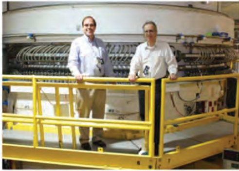
▲ Paul Brand and Tony Norbedo (l-r) celebrate the start of commissioning by the ring header of the newly installed thermal shield system.
