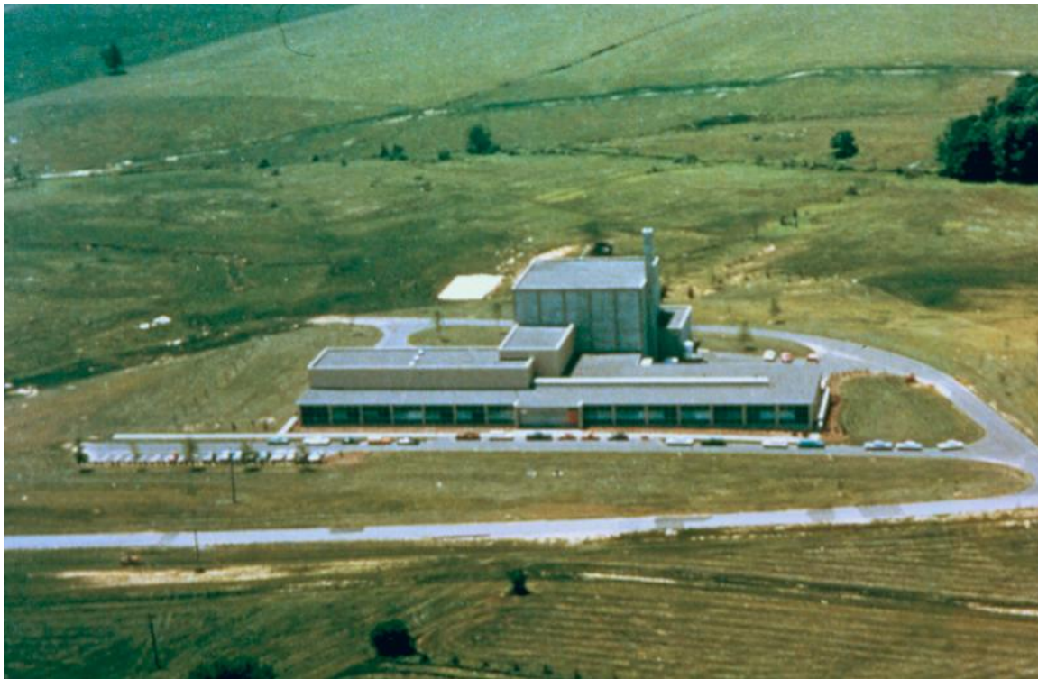
An aerial view of the NBS reactor confinement building (at the rear) and the original office and laboratory buildings, circa 1970.
