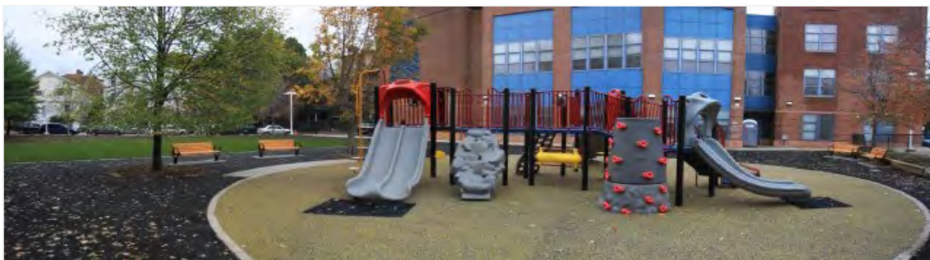
Pictured: Haynes Early Education Center schoolyard improvements
