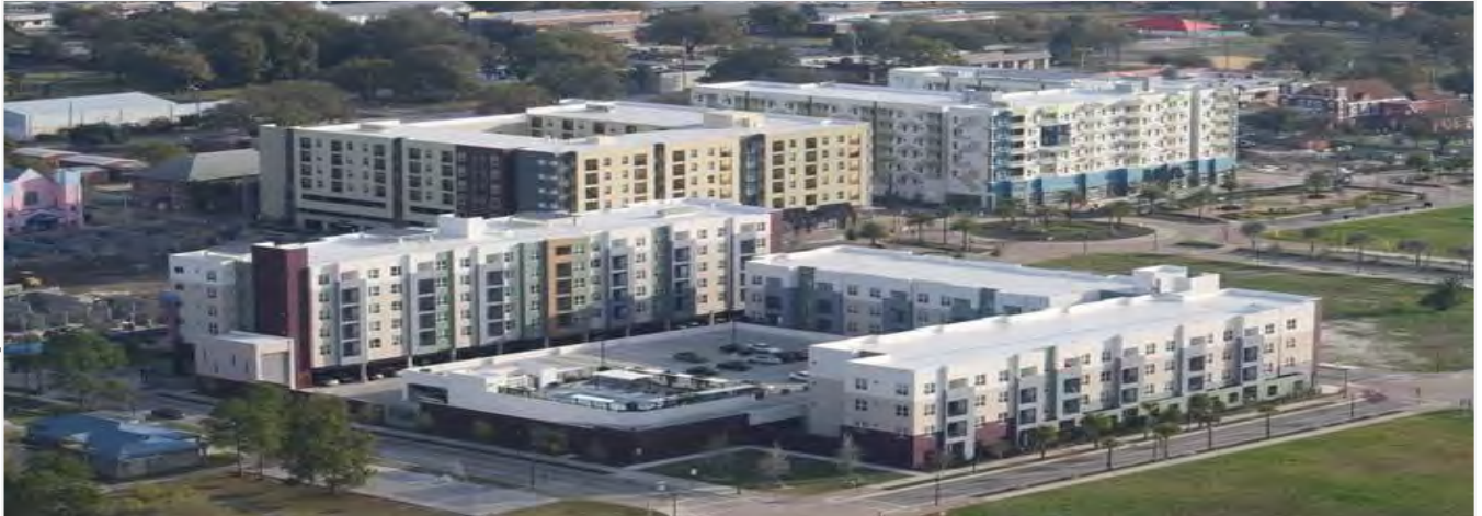
Pictured: Aerial view of development completed and underway within Encore
