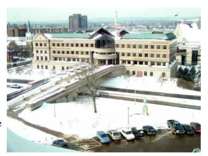
The five-story building was built along the enclosed Park River and is supported by pilings sunk 50 feet into the earth.
