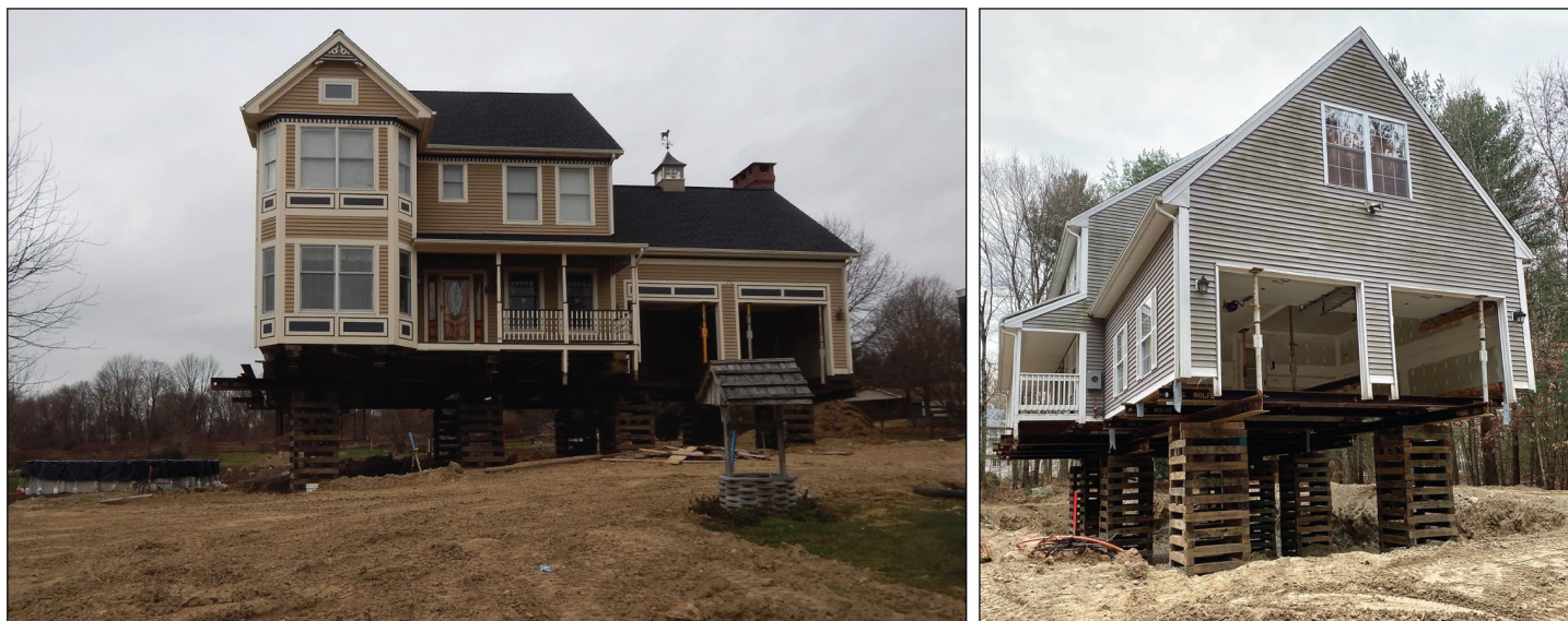
Figure 4: Homes Elevated to Replace Pyrrhotite-Damaged Foundations
