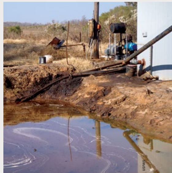
Spilled oil at a production facility at Lake Ophelia National Wildlife Refuge in Louisiana.
