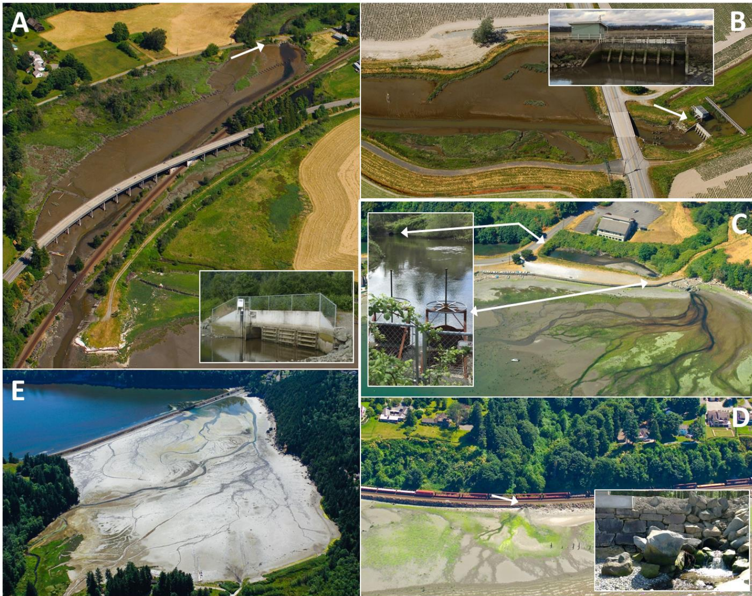
Figure 1. Examples of intertidal water crossing structures in Puget Sound WA. A. Railroad and highway bridges, road grades, dikes on the seaward boundaries, and tidegates including a tidal muting structure (see inset of road crossing denoted by arrow) at McElroy Slough at the north end of Samish Bay. B. Dikes and road crossings surround Big Indian Slough in Padilla Bay. A set of culverts with flap-style tide gates (inset) is located at the arrow. C. Open culverts (at arrows and in inset) under road crossings drain a lagoon in Port Susan. D. Railroad grade between Everett and Mukilteo that crosses a coastal creek confluence with a culvert (inset and arrow). E. Chuckanut Bay south of Bellingham, dissected by a railroad causeway with bridge. Landscape images are from the WA Coastal Photo Atlas. Inset photo credits: A. Brittany Jones, B. Eric Beamer, C. Correigh Greene, D. Jason Hall.
