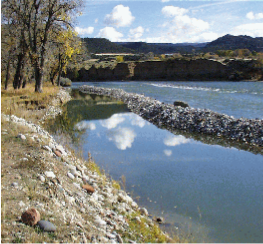
The Silt Diversion before improvements
