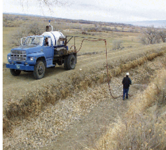
In 2000 the Uncompahgre Valley Water Users sprayed a polyacrylamide solution on 13 miles of canals and laterals as part of a canal sealing demonstration.
