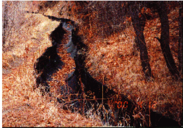
An installed reach of "Fast Ditch" ditch liner
