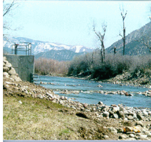
The improvements to the Silt Diversion were completed in FY2000
