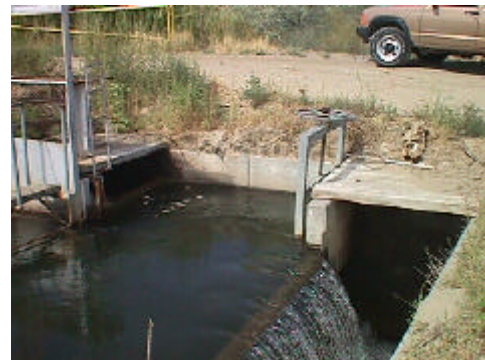
One of four key spill sites to be measured on the Hammond Main Canal.
