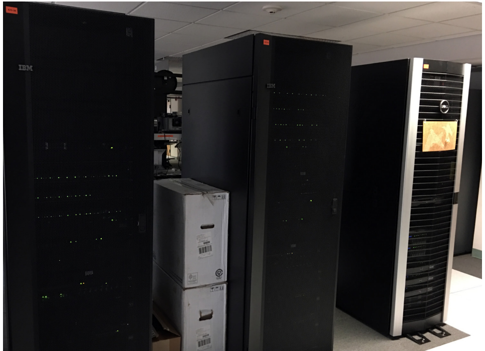
Figure 7: National Weather Service Telecommunication Gateway Server
