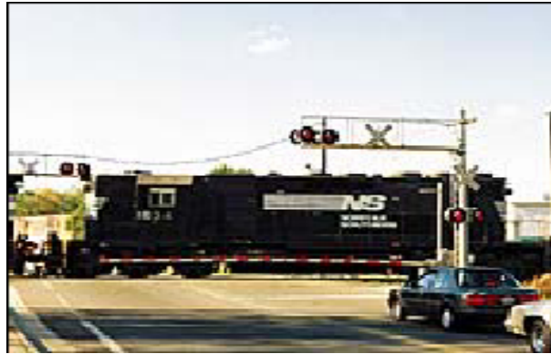
Figure 6: Grade Crossing with Long Gate Arm
