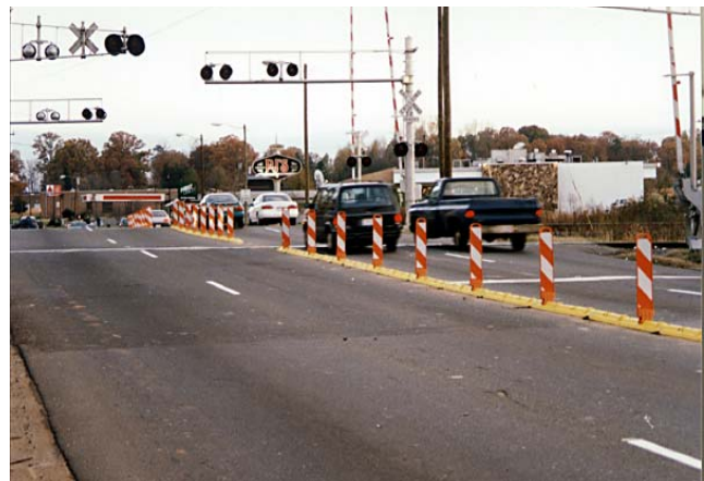
Figure 5: Grade Crossing with Flexible Traffic Channelization Devices
