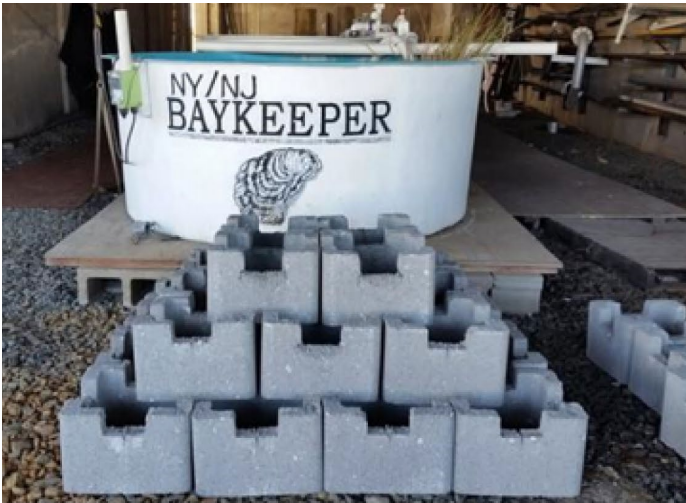
An oyster castle before being placed in the water to form a living reef that can dissipate wave energy and reduce waves' storm impacts.
