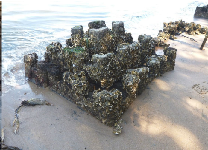
A populated oyster castle similar to those at Naval Weapon Station Earle, New Jersey, from a project in Virginia.
