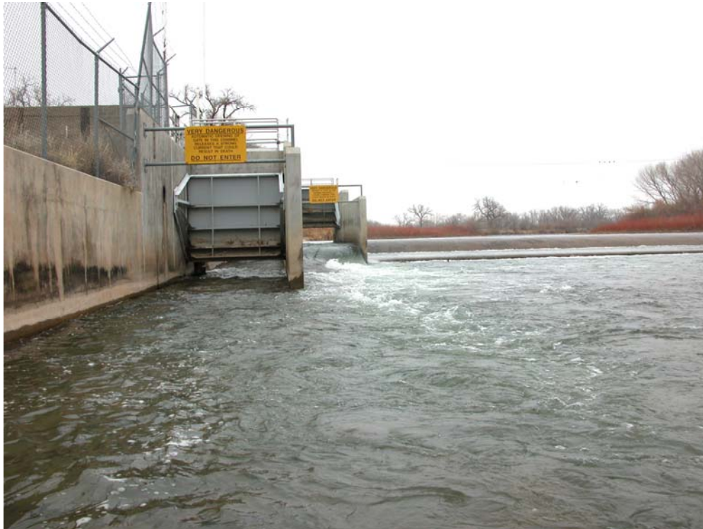
Figure 2: City of Farmington's Animas Pump Station #2 (APS) with open gates.
