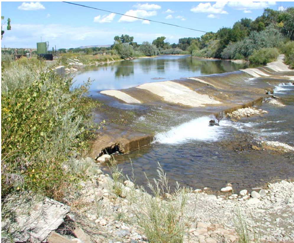
Figure 3: Farmer's Ditch Diversion (FDD) at relatively low flow conditions.
