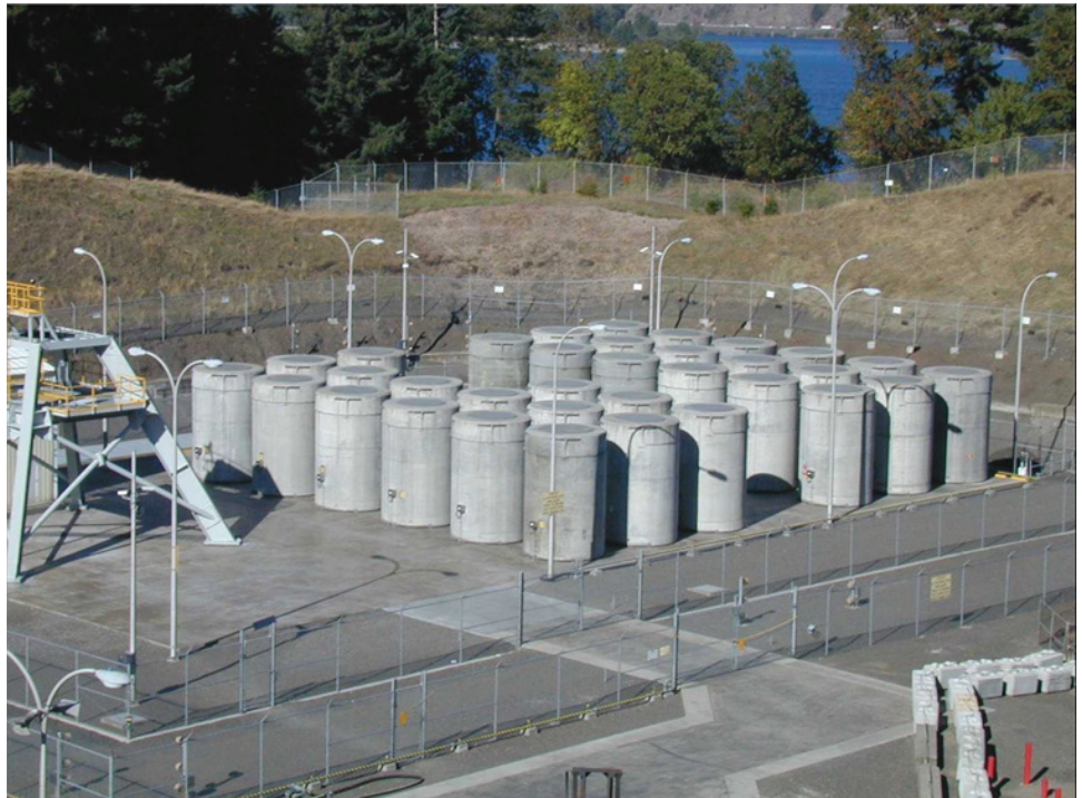
Figure 2: Spent Nuclear Fuel Stored in Dry Casks at the Trojan Independent Fuel Storage Installation in Oregon
