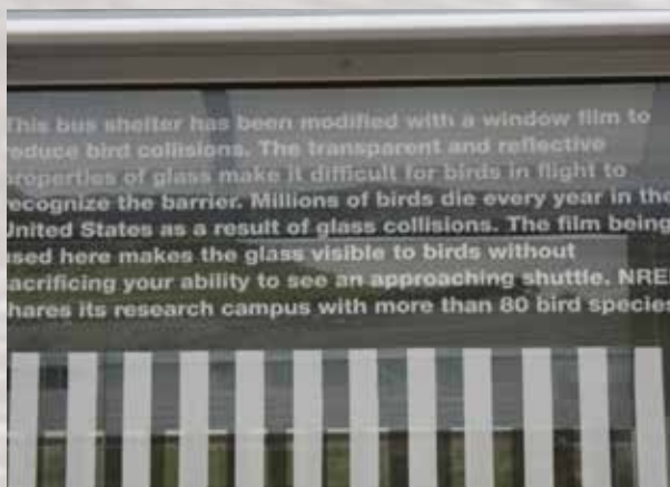
Bus shelter at DOE’s National Renewable Energy Lab retrofitted with Colidescape to reduce bird strikes. Photo Credit: National Renewable Energy Lab, DOE
