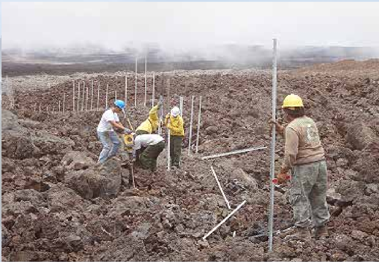
Predator fence construction at Hawai'i Volcano National Park. Photo Credit: National Park Service.
