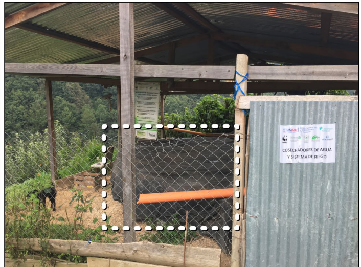
Rainwater reservoir used by a farmer to store water from the rainy season for irrigation during the dry season and during the canicula (the dry period during the rainy season).
