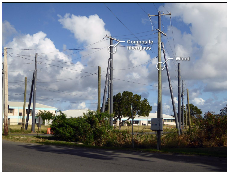
Figure 12: Wooden and New Composite Fiberglass Utility Poles in St. Croix, U.S. Virgin Islands
