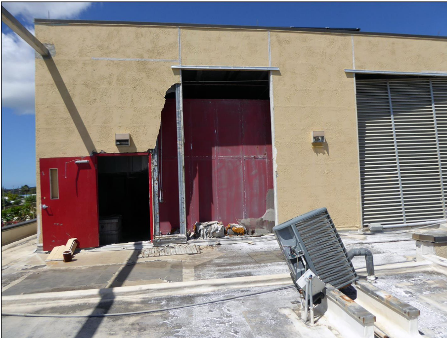
A section of the facility that was sheared off during the hurricane leaving the building's ventilation units susceptible to outdoor conditions.
