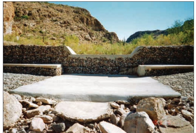
Figure 9. The reconstructed fish barrier on Arnett Creek, Pinal County, Arizona.
