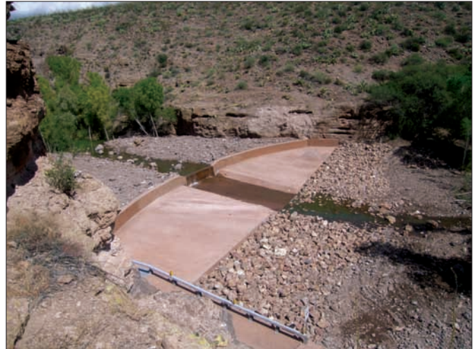
Figure 5. The fish barrier on Bonita Creek, Graham County, Arizona.
