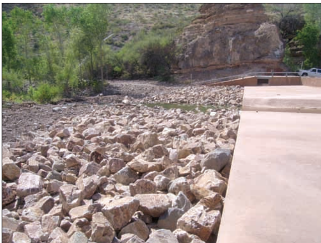
Figure 3. Riprap placement downstream from the apron of the Bonita Creek fish barrier, Graham County, Arizona.
