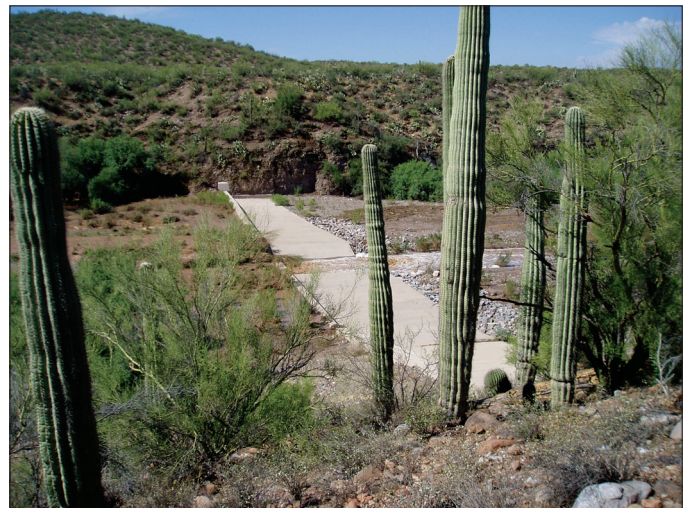
Figure 6. The lower fish barrier on Aravaipa Creek, Pinal County, Arizona.
