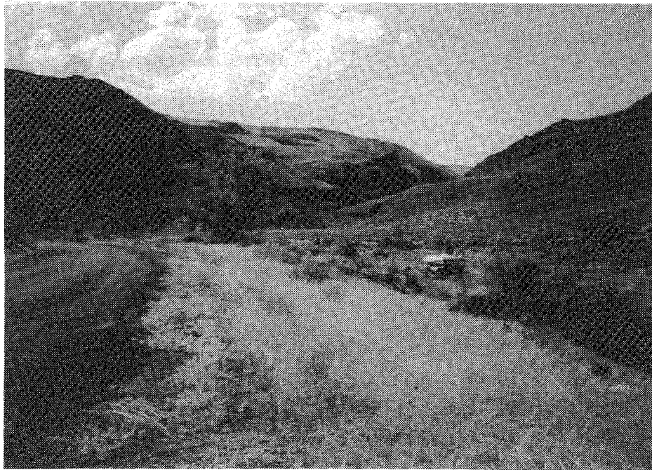
Photo 3-19: Site D. Access to many sites, including Site D, is steep, causing erosion and potential safety problems.
