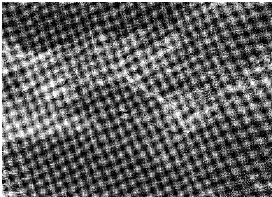
Photo 3-25: Malheur County Boat Ramp. The one-lane boat ramp is steep and narrow.
