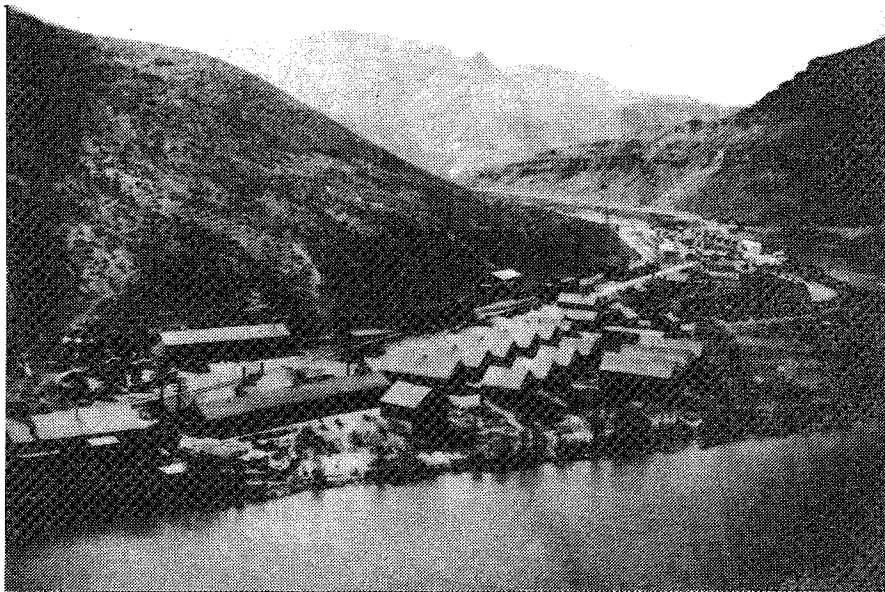
Photo 3-9: Contractor’s Camp at Owyhee Damsite. During 1928, a contractor’s camp for employees of the General Contracting Company was erected between Government Camp and the damsite.
