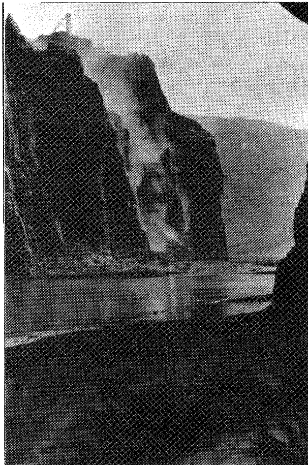
Photo 1-2: Stripping East Canyon Wall of Loose Rock. Photographic copy of historic photo, September 22, 1928.
