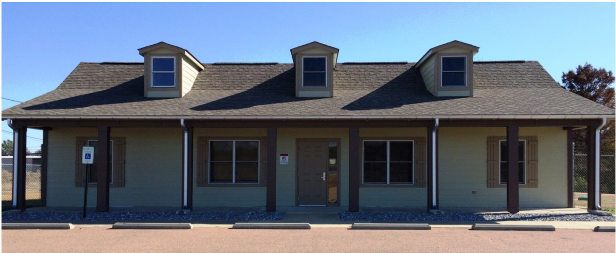
Rehabilitated headquarters building at Morgan Brake NWR, MS.
