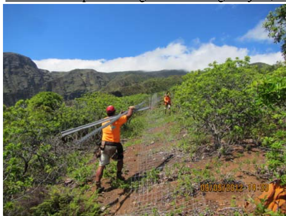
Fence construction crew on Molikai Island, HI
