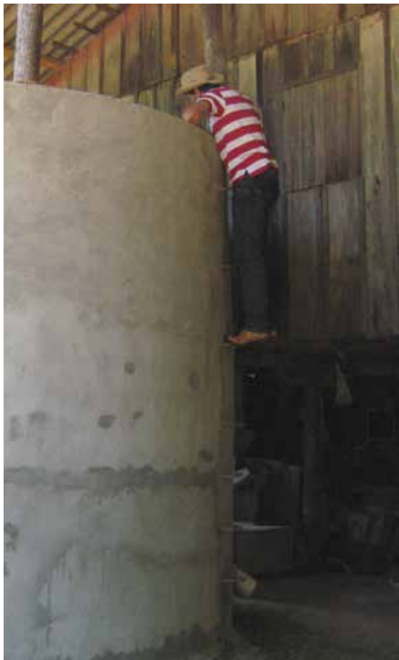
Inspecting a cistern.
